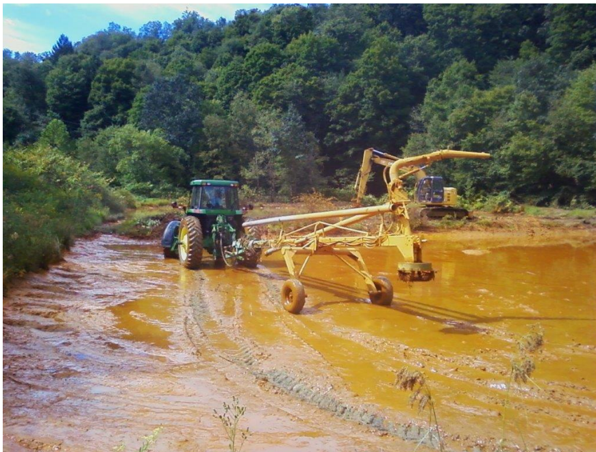
Photo 6. Sludge pumping equipment used for the Wolford project. The pond has been drained down and much of the sludge already removed. The photo shows the pump being moved.
