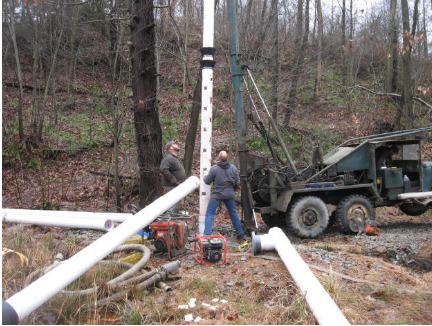
Photo 1. Perforated pipe and shale traps being lowered into the borehole
