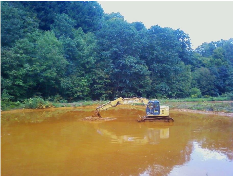
Photo 8. Sludge was pushed toward the pumping station using an excavator.
