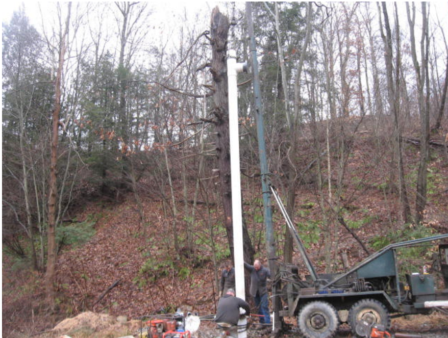
Photo 2. Solid pipe being lowered into the borehole
