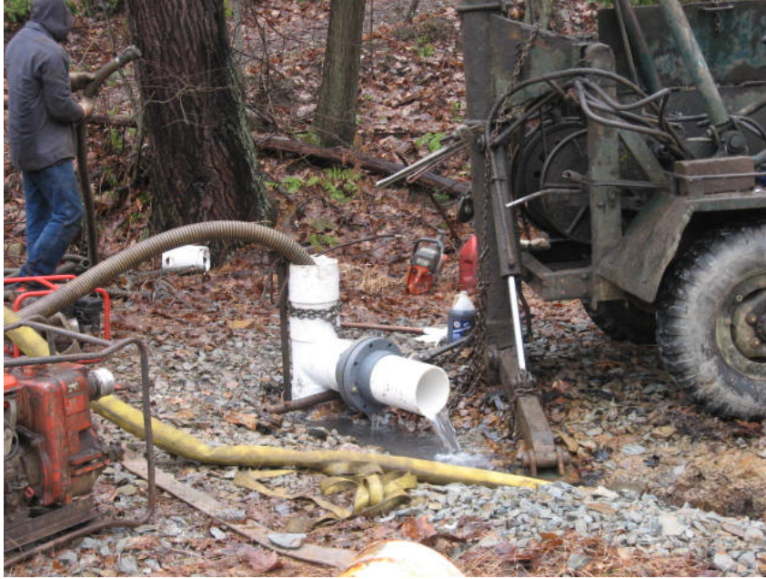
Photo 3. Finished pipework with grout injection
