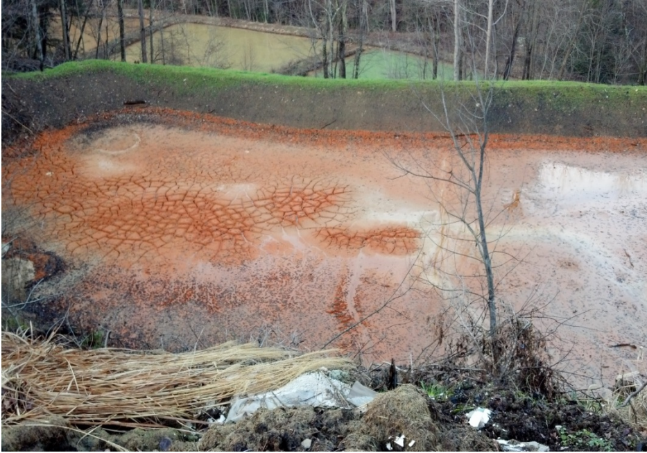
Photo 9. The sludge basin in December 2012. The sludge dewatered naturally in place (note the cracking) and then was stacked in small piles to promote drying.
