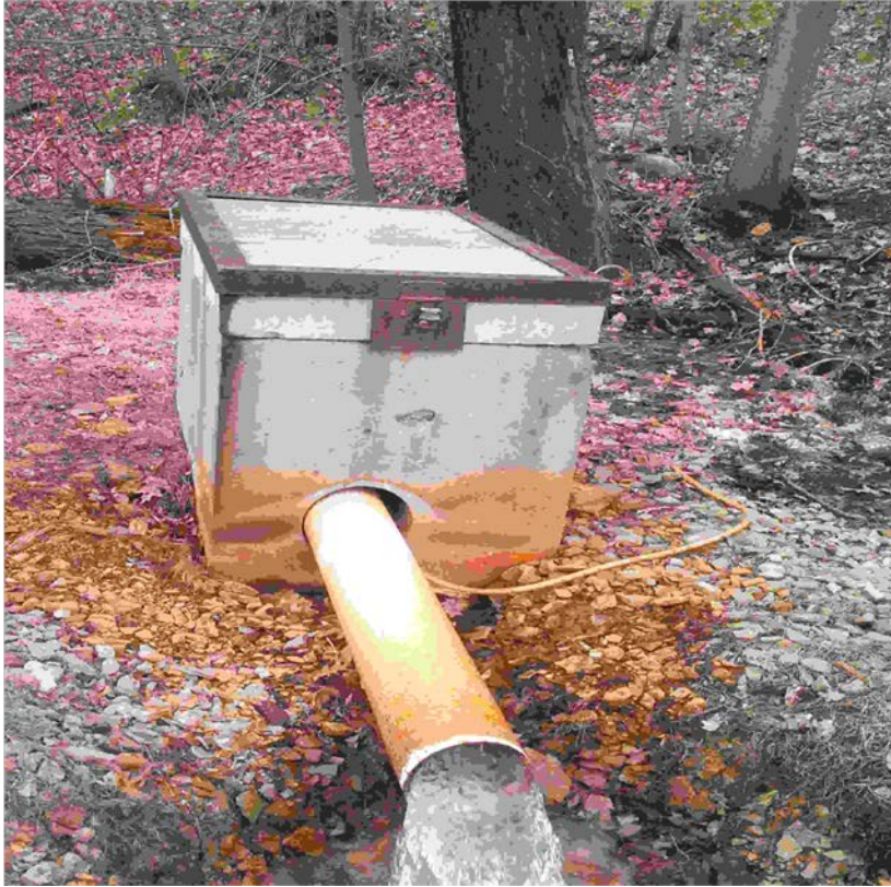
Photo 5: Concrete Vault Protection of Wolford Borehole Improvements.
