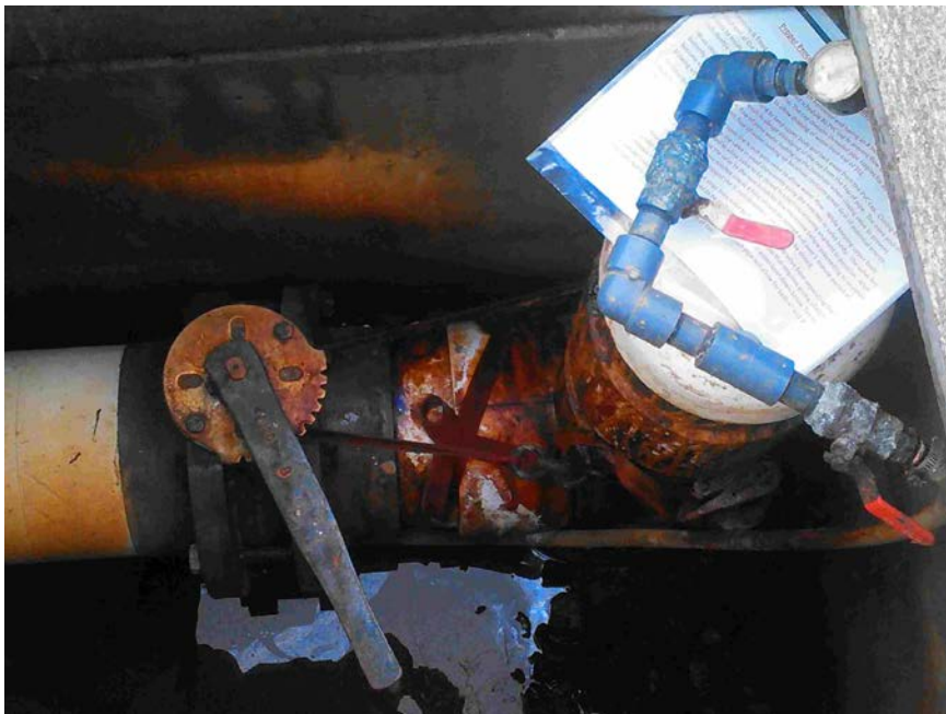
Photo 4: Wolford Borehole Improvements.
