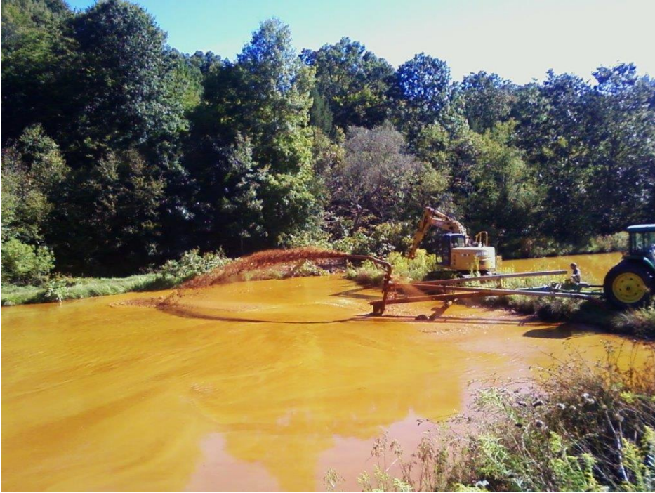
Photo 7. Sludge pump in operation at Wolford. The pump both mixes (spraying) and pumps. The photo shows mixing operation.
