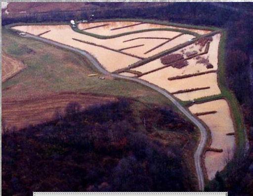
Aerial Photograph of Wetland #1
