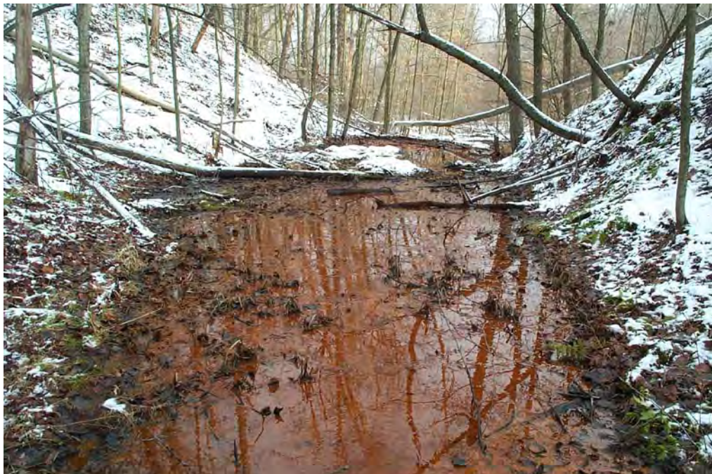
The SR96 discharge flowing through the spoil breach.
