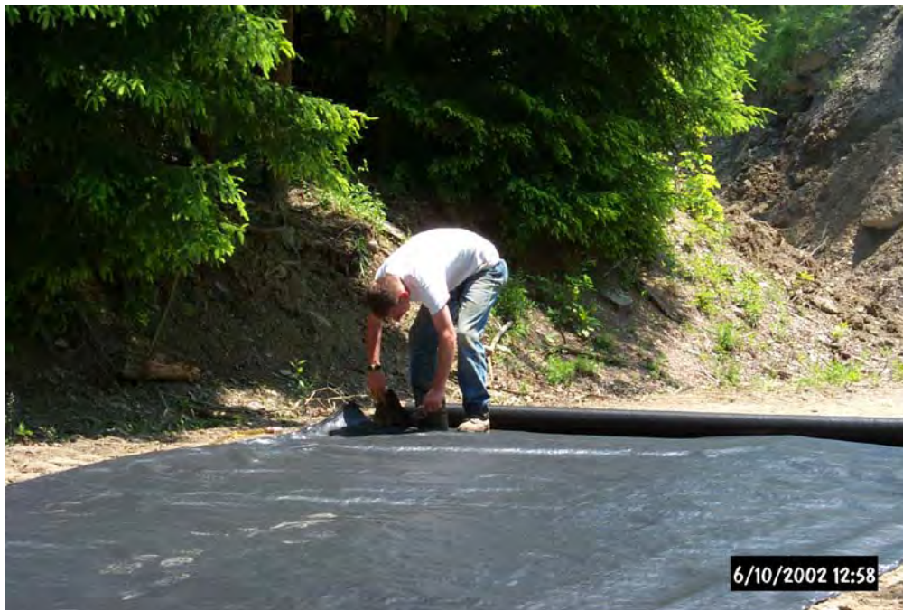
Jason Jesteadt installing the geotextile fabric before the limestone is placed.
