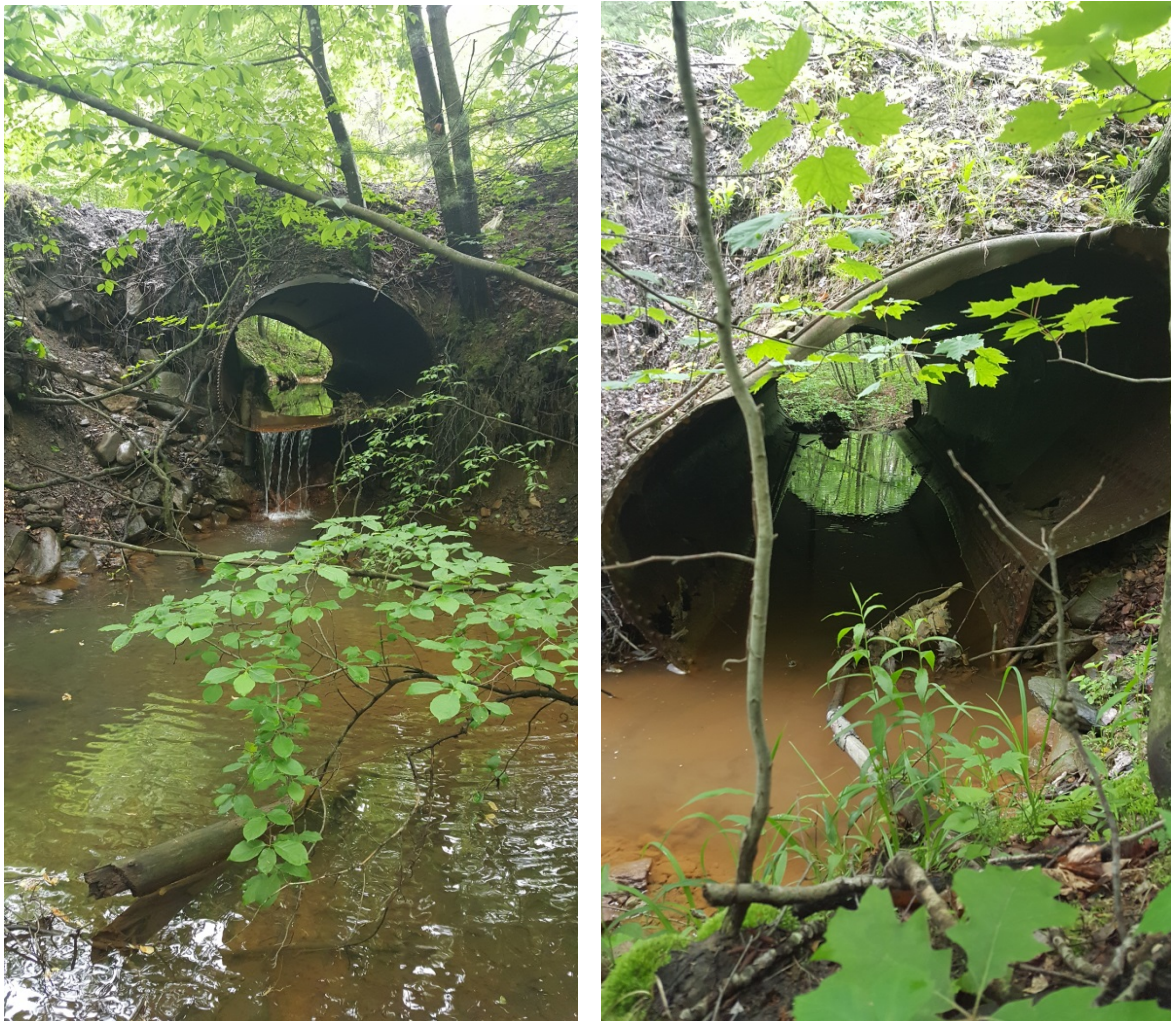
Figure 5 a & b: Deformation, outlet drop, and erosion around culvert at site CR01 downstream (a) and deformation and erosion around pipe upstream (b).
