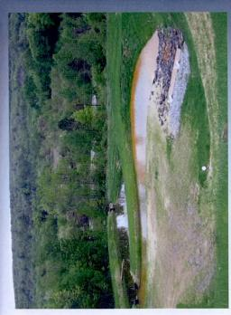
the water are then able to precipitate or drop out of the water into two wetland cells after leaving the OLD. This allows the metals to be pollution entering the Wabash Creek and the Little Schuylkill River and provides habitat for various species of wildlife. removed from the water and the pH to be increased before the water reaches the Wabash Creek. The project is reducing the amount of
