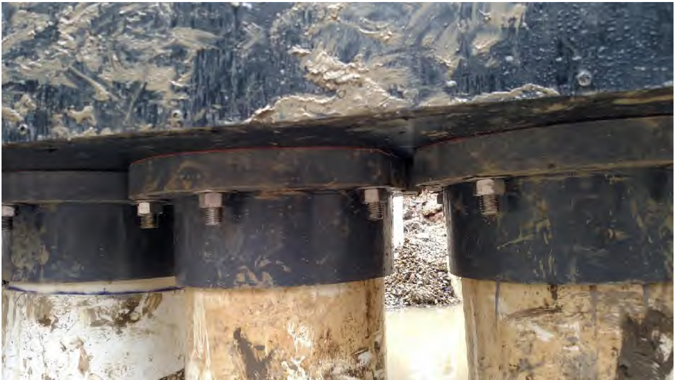
Top: Trompe outlet weir box with trompe inlets and splitter box in the background. Bottom: Up-close of the trompe uppipes plumbed into the bottom of weir outlet box.
