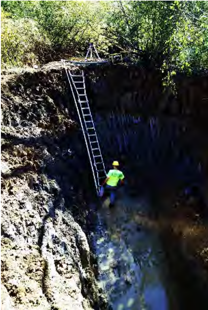
Left: Confirming proper elevations in the excavation before trompe installation Right: Lowering the 14" diameter trompe separation chamber into the ground
