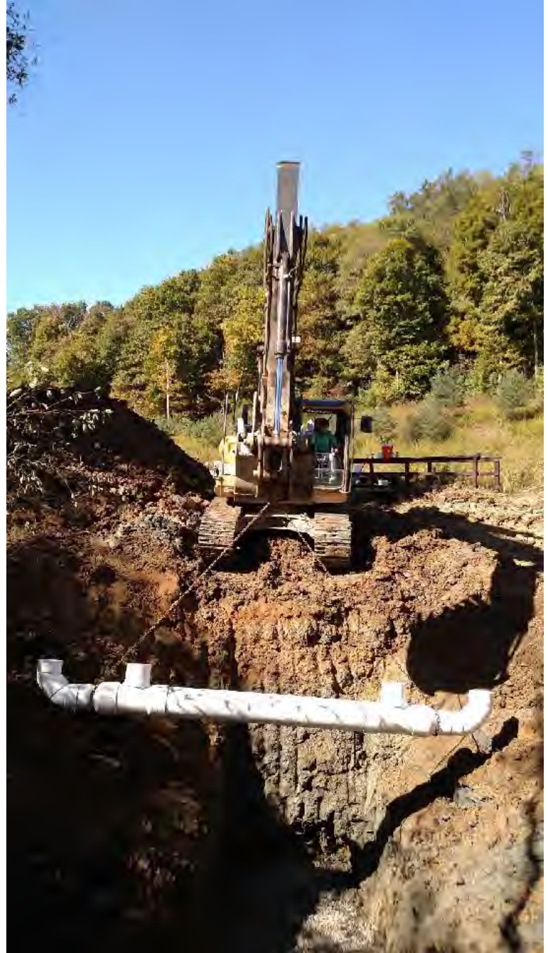
Left: Confirming proper elevations in the excavation before trompe installation Right: Lowering the 14" diameter trompe separation chamber into the ground
