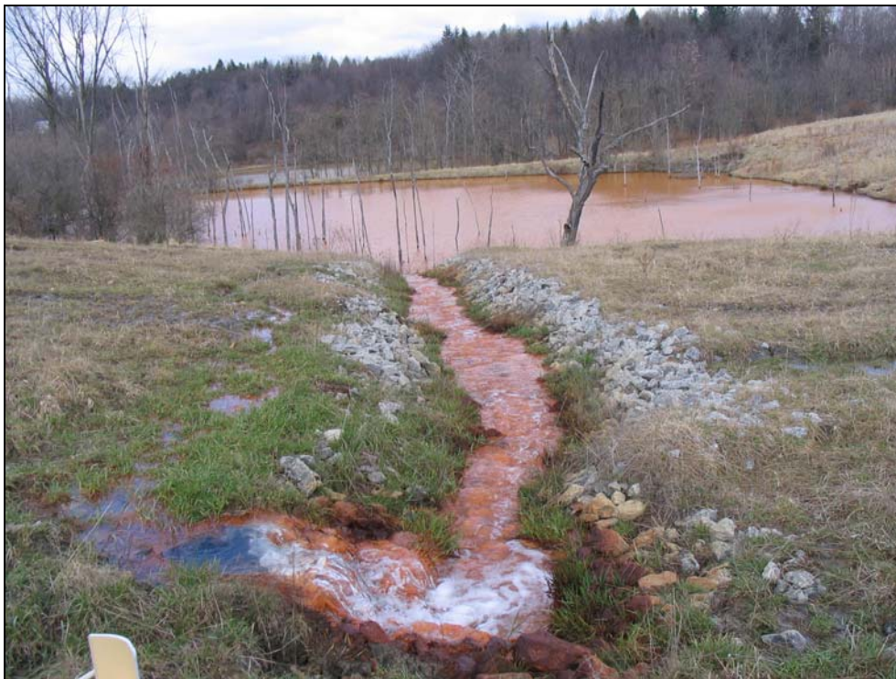
Photo A. The discharge from the ALCD and its flow down the ditch into Pond 1.
