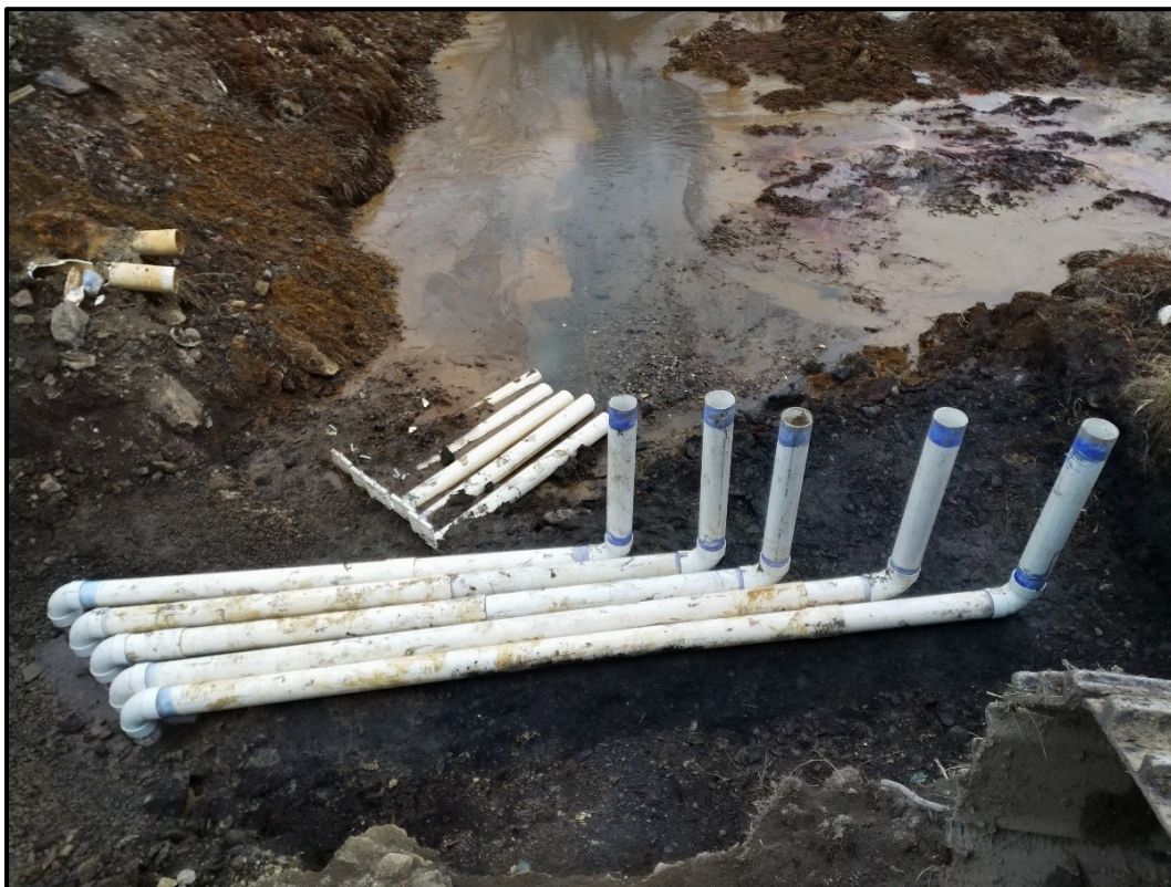
Top: JVFP3 outlet pipe installation (8/6/20).
