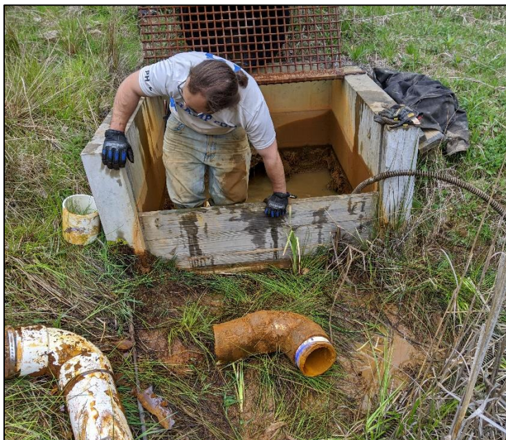
Top Left: Excavation near the VFP-N outlet pipe revealed there was a break (2/19/20).
