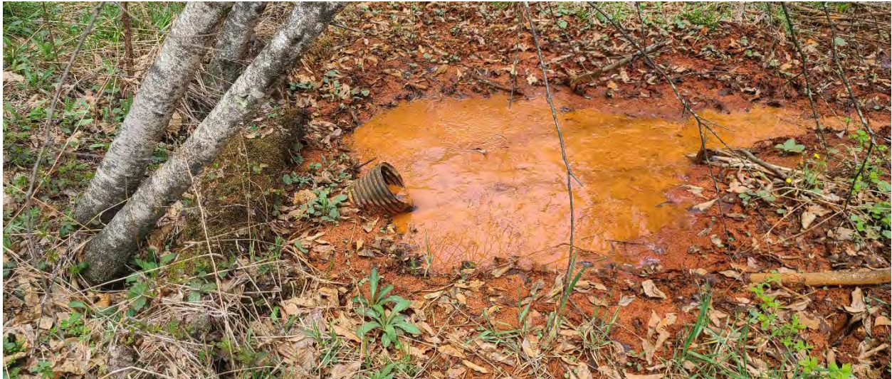
Top: Pre-rehab photo of Wetland D2 (WL D2). After 26 years of operation the component was filled with iron precipitates and vegetation. (2021)
