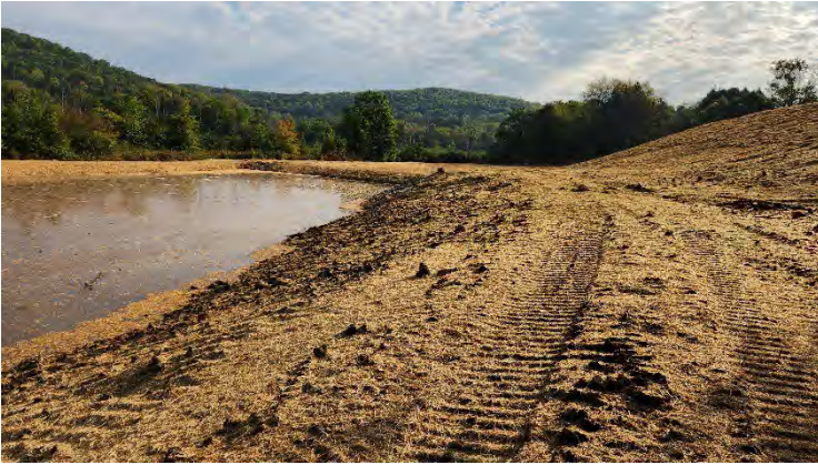
Top Photo: Cleaned settling pond (left), ALD 2 after placement of cover material (center), and ALD 1 prior to installation of new limestone (right). (2023)
