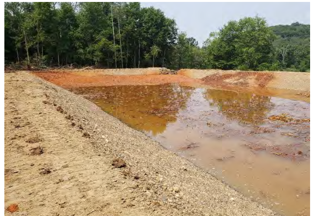
Top Left: Construction of the dewatering basin to hold sludge and debris removed from the SR81 settling pond and wetland. (2023)
