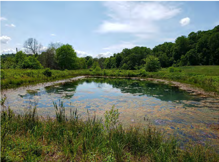
Top Left: Pre-rehabilitation photo of VK2 (JVFP West), the limestone-only vertical flow pond that followed VK1. Due to clogging issues of VK1, the water was directed to bypass the VK1 treatment media and enter directly into VK2 until rehabilitation could take place. The Agri Drain outlet structure (foreground) had numerous stop logs stuck and was no longer fully operational. (2020)
