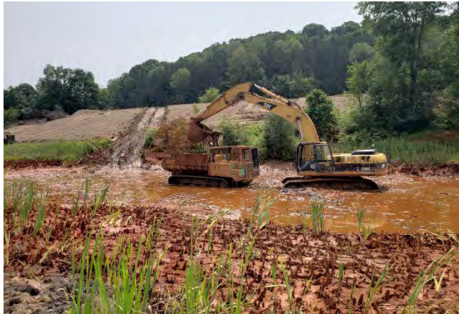
Top Left: Construction of the dewatering basin to hold sludge and debris removed from the SR81 settling pond and wetland. (2023)
