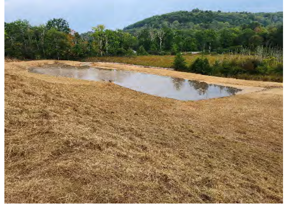
Top Photo: Cleaned settling pond (left), ALD 2 after placement of cover material (center), and ALD 1 prior to installation of new limestone (right). (2023)
