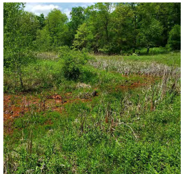
Above Photos: After 22 years of operation, the ponds and wetlands of the SR101A treatment system were essentially filled with iron precipitates. The system has functioned as intended by preventing the iron from entering Slippery Rock Creek. (2020)
