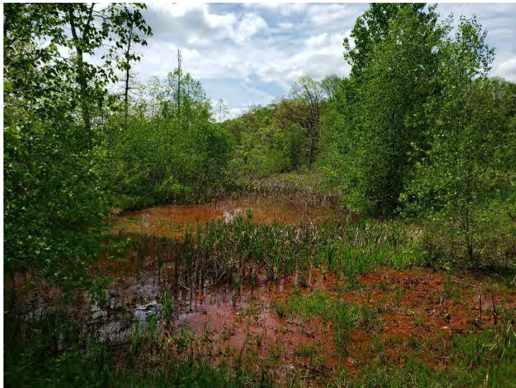
Above Photos: After 22 years of operation, the ponds and wetlands of the SR101A treatment system were essentially filled with iron precipitates. The system has functioned as intended by preventing the iron from entering Slippery Rock Creek. (2020)
