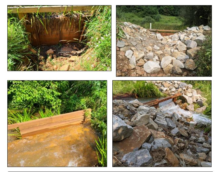
Top Left: Pond 10 overflow weir eroded on downstream side (7/2/21).
