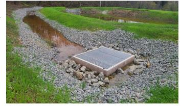
After Rehabilitation: Terraced iron formation (TIF) and flow splitter box at the Ferris SR85/86 passive system with the JVFP East (VK1) in background.
