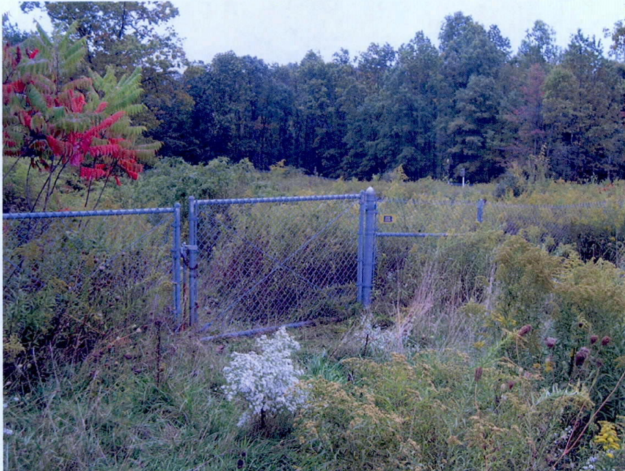
Access gate and fencing around treatment ponds. Date of Photo: 10-2-08.
