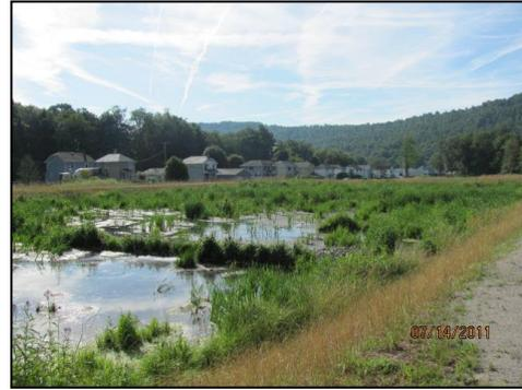
*The aerobic wetland section of the Melcroft Treatment System*
