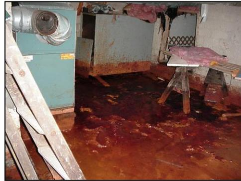
*Mine drainage backing up into the basement of a home before the construction of the Melcroft Treatment System*
