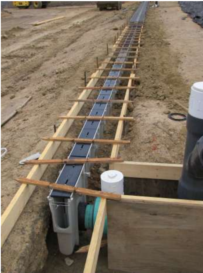
Photo 18: Treatment cell intake piping and trench drain construction.
