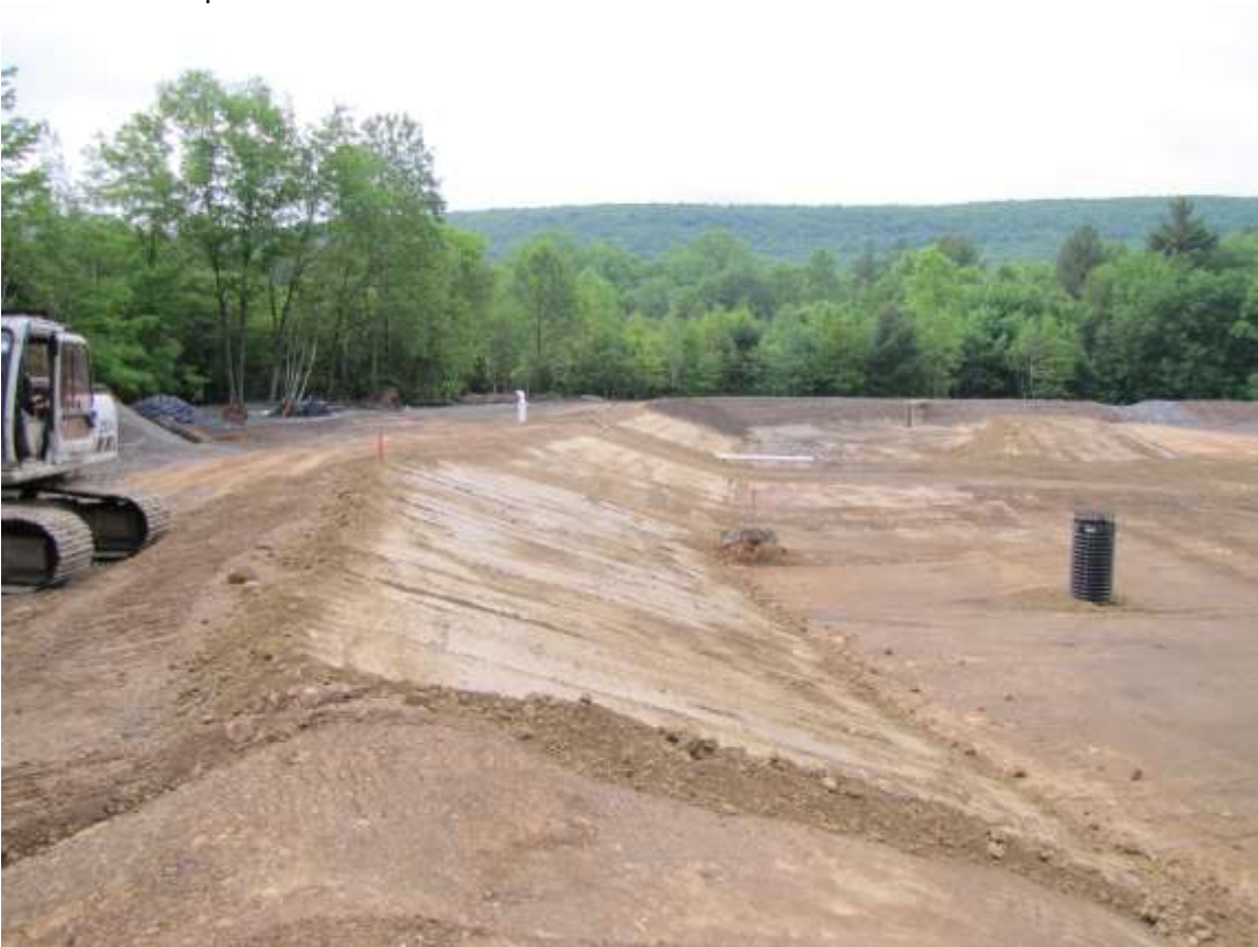
Photo 22: Nearly complete settling pond showing the intake riser, dry hydrant, water level control structure and drain and emergency spillway.
