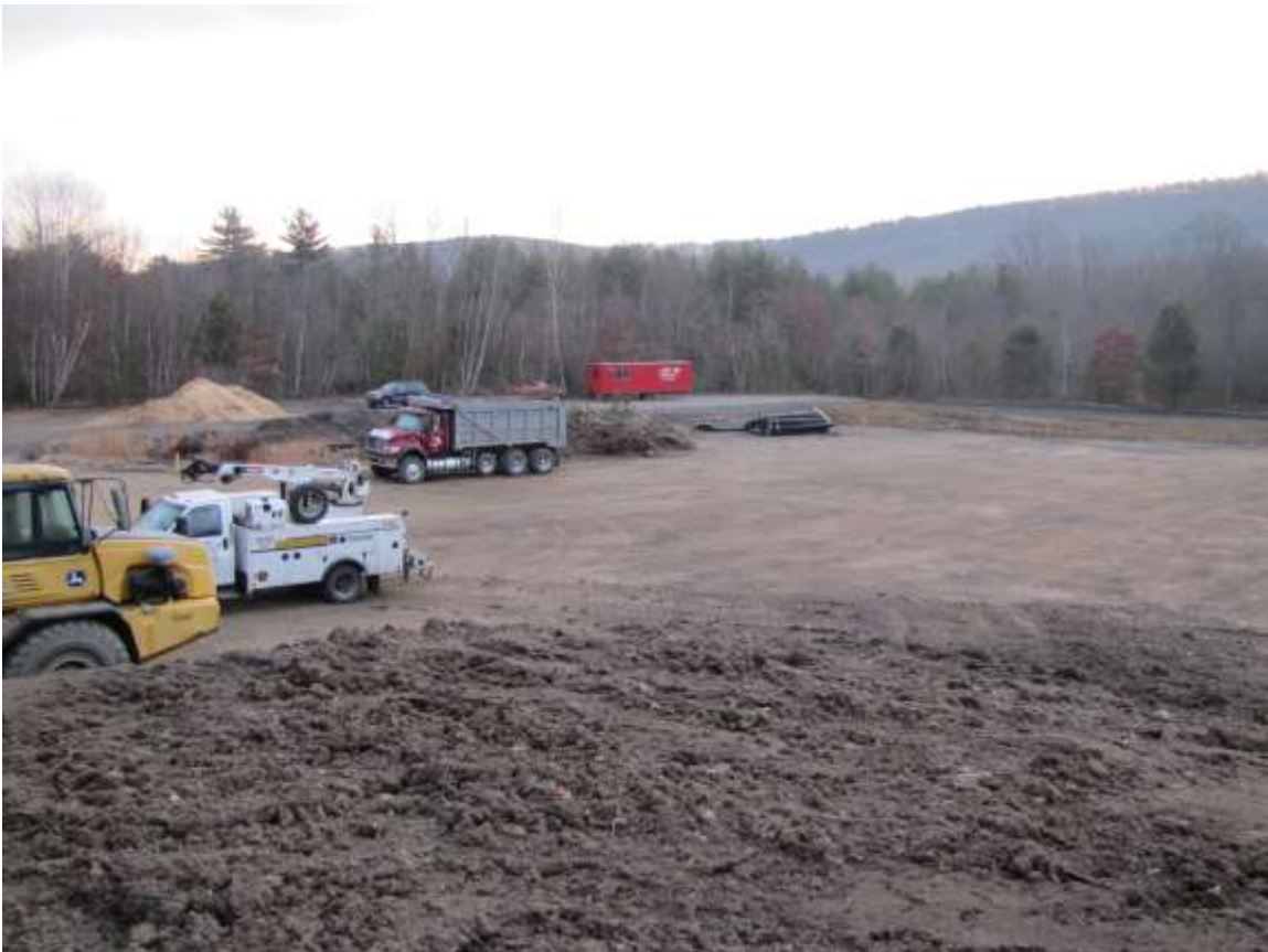
Photo 6: Beginning of construction of treatment system.
