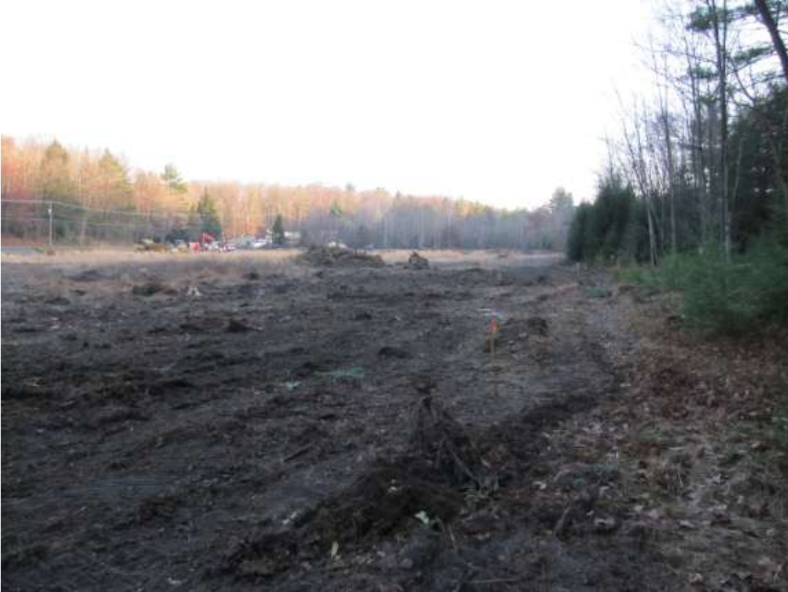
Photo 4: Topsoil stripping of project site for construction of treatment system.
