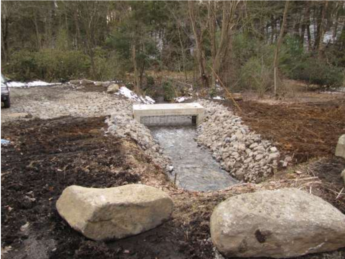
Photo 11: Completed intake structure by-passing 100% of the borehole flow.
