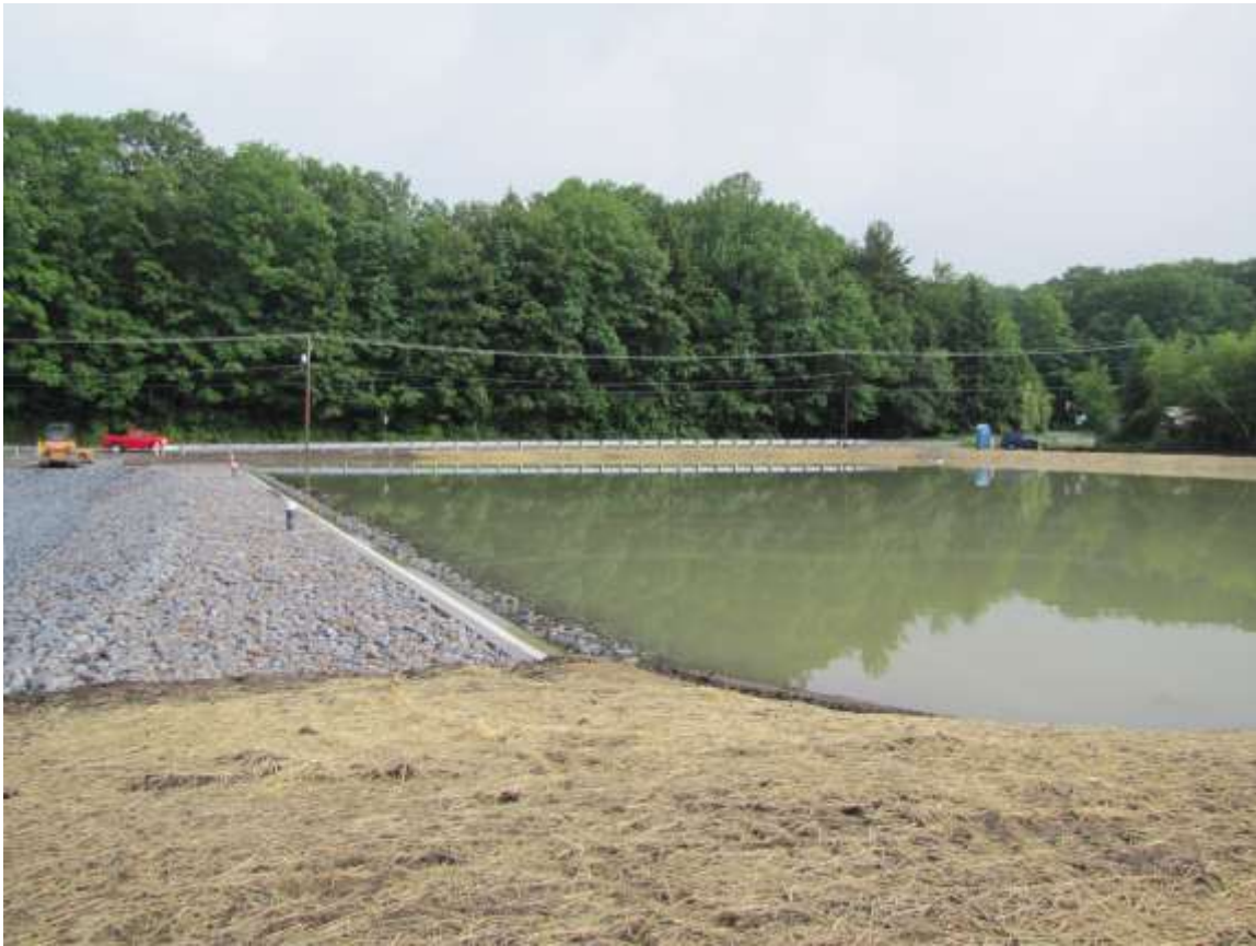
Photo 25: Settling pond and wetland cell filled.
