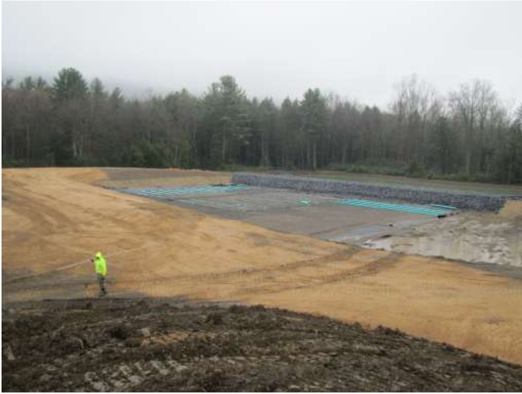
Photo 17: Piping placement in the bottom of the treatment cell.
