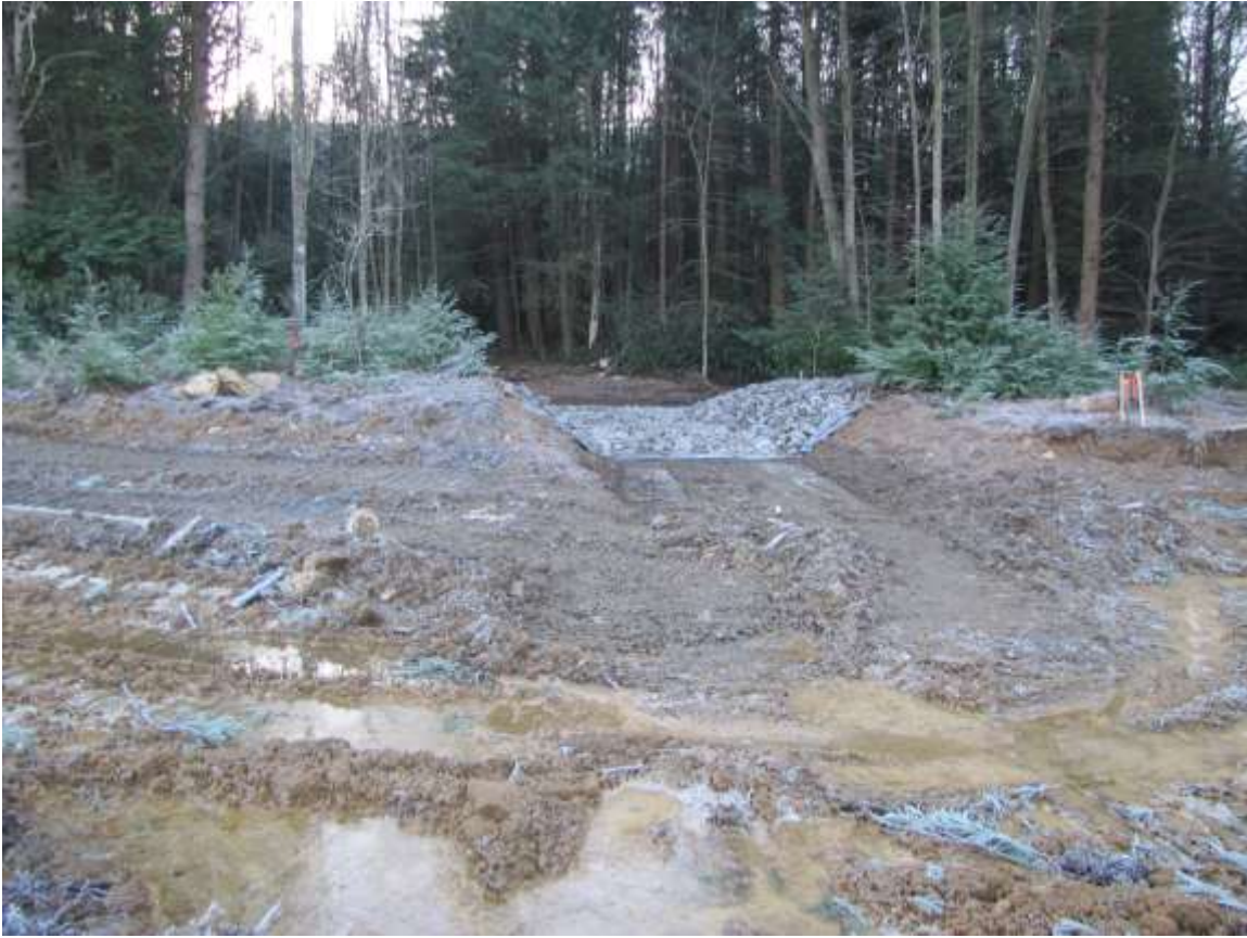
Photo 5: Construction of limestone rip-rap emergency spillway to the Schuylkill River.
