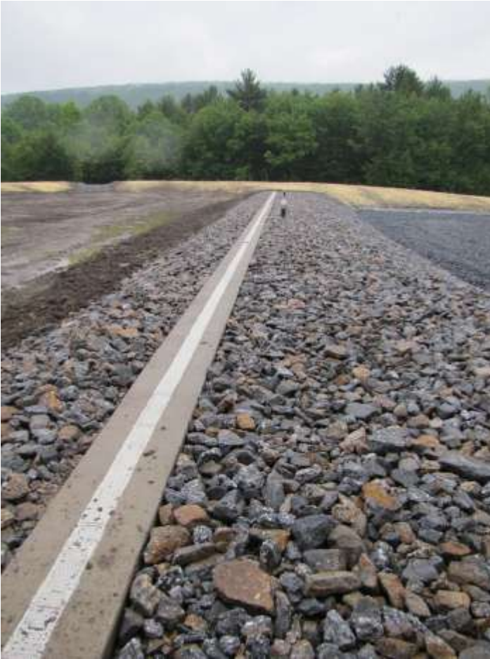
Photo 19: Completed trench drain and treatment cell intake system.
