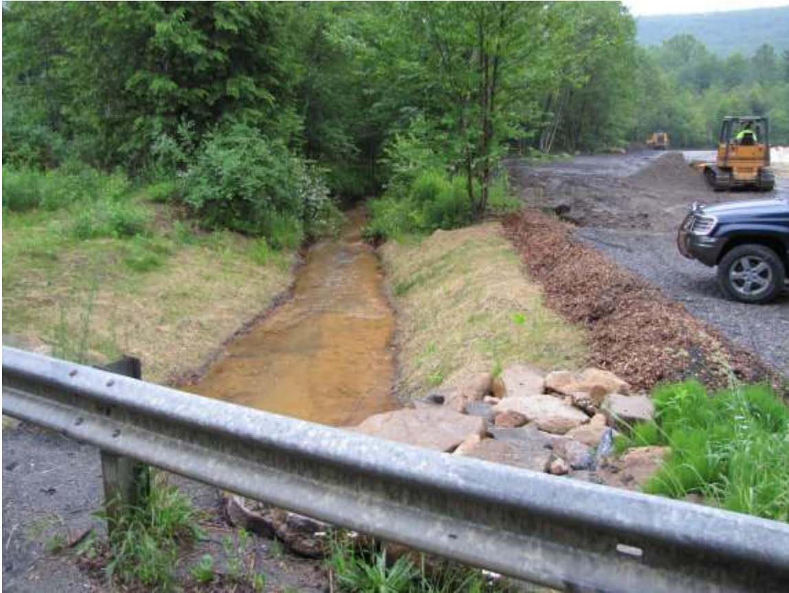
Photo 13: Completed stream crossing.
