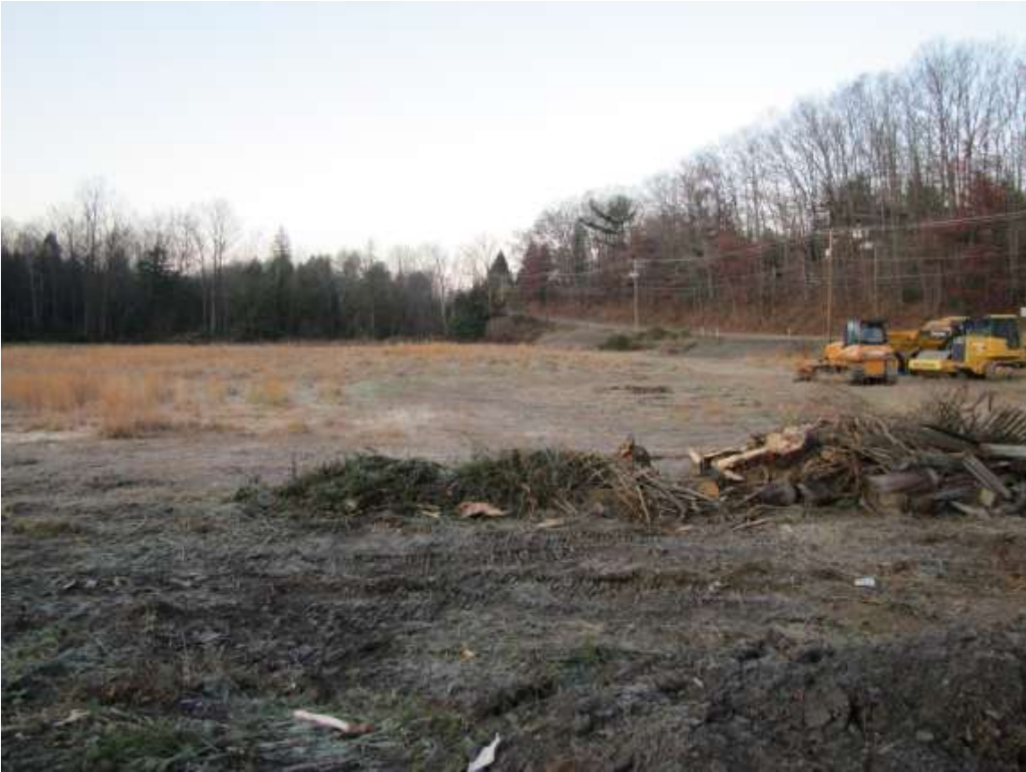
Photo 3: Clearing & grubbing of the project site.
