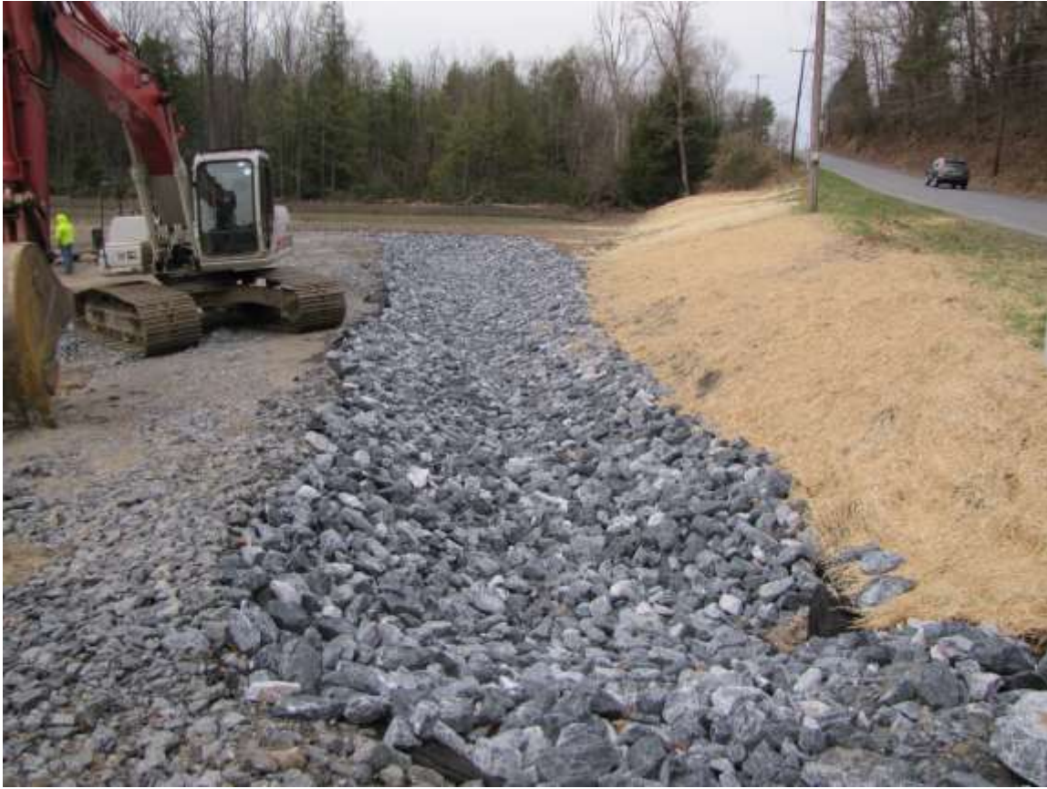
Photo 15: Outfall channel tie-in to existing roadway culvert.
