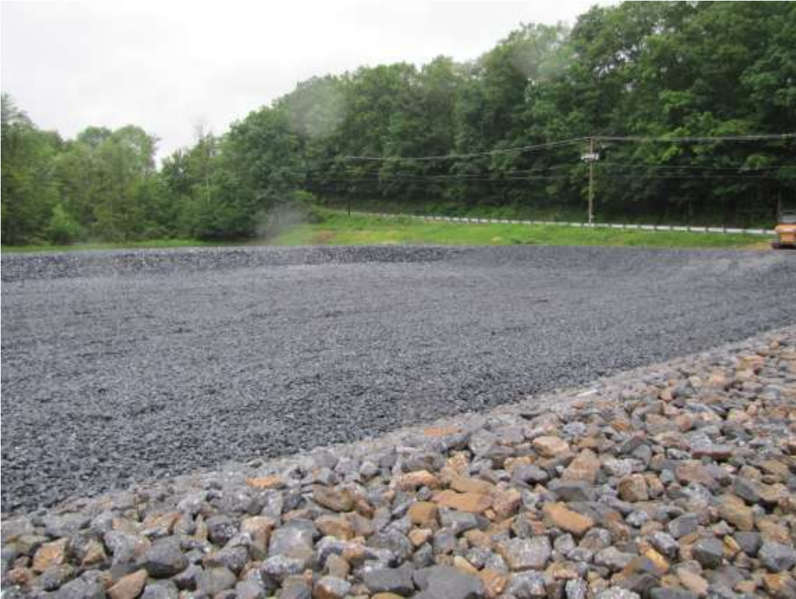
Photo 21: Completed treatment cell.
