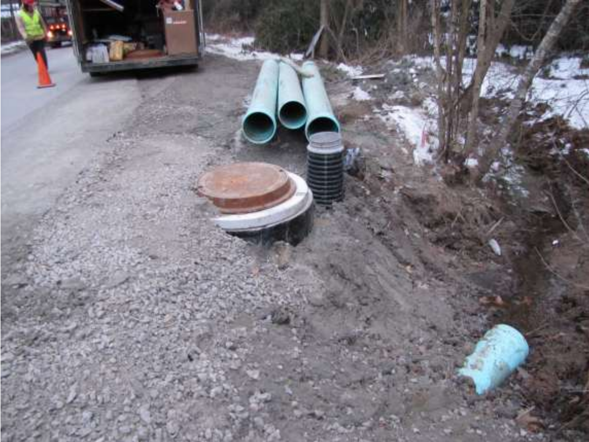
Photo 8: Installation of intake piping from the mine borehole beside Twp. Road 505.
