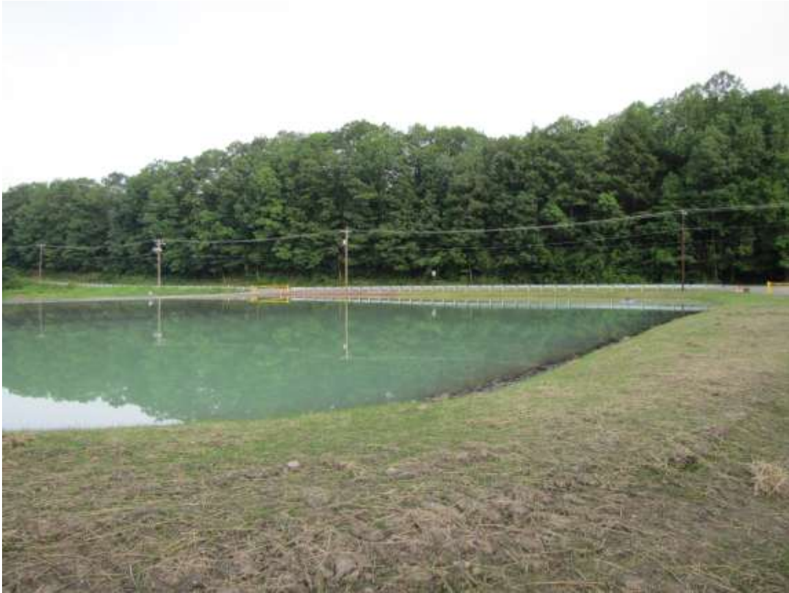
Photo 29: Completed seeding and mulching of entire project site.
