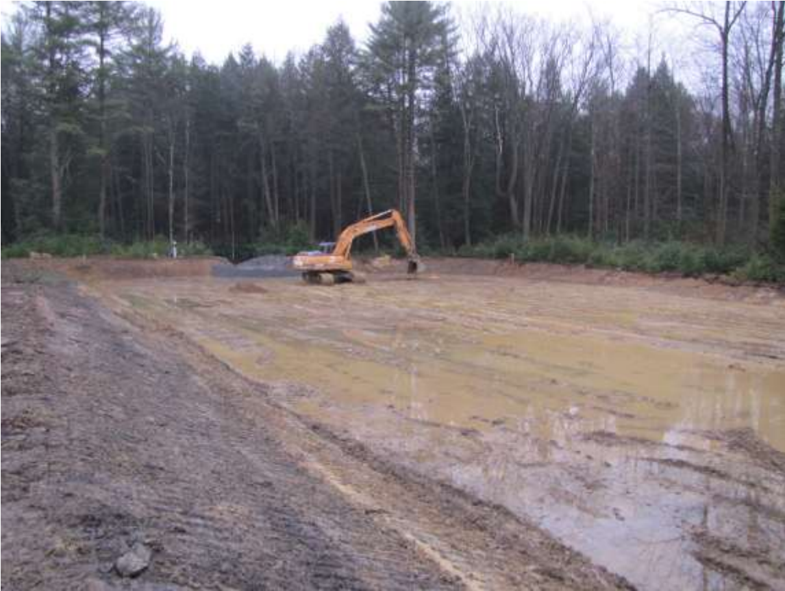
Photo 7: Construction of flushing pond south of the treatment cell.
