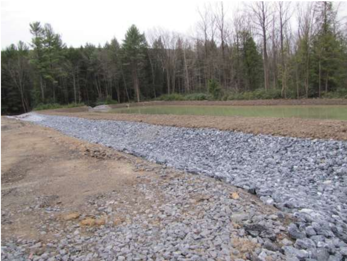
Photo 14: Outfall channel to Schuylkill River with flow measurement weir in background.
