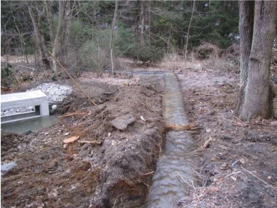
Photo 9: Installation of intake structure and temporary by-pass of borehole discharge.
