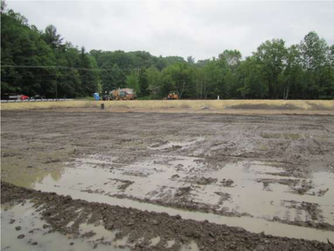
Photo 23: Completed settling pond and wetland cell.
