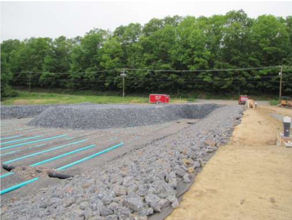
Photo 20: Treatment cell limestone addition.
