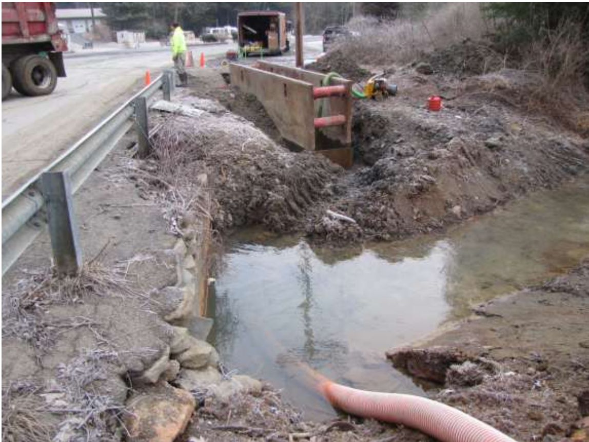
Photo 12: Preparing for the stream crossing.
