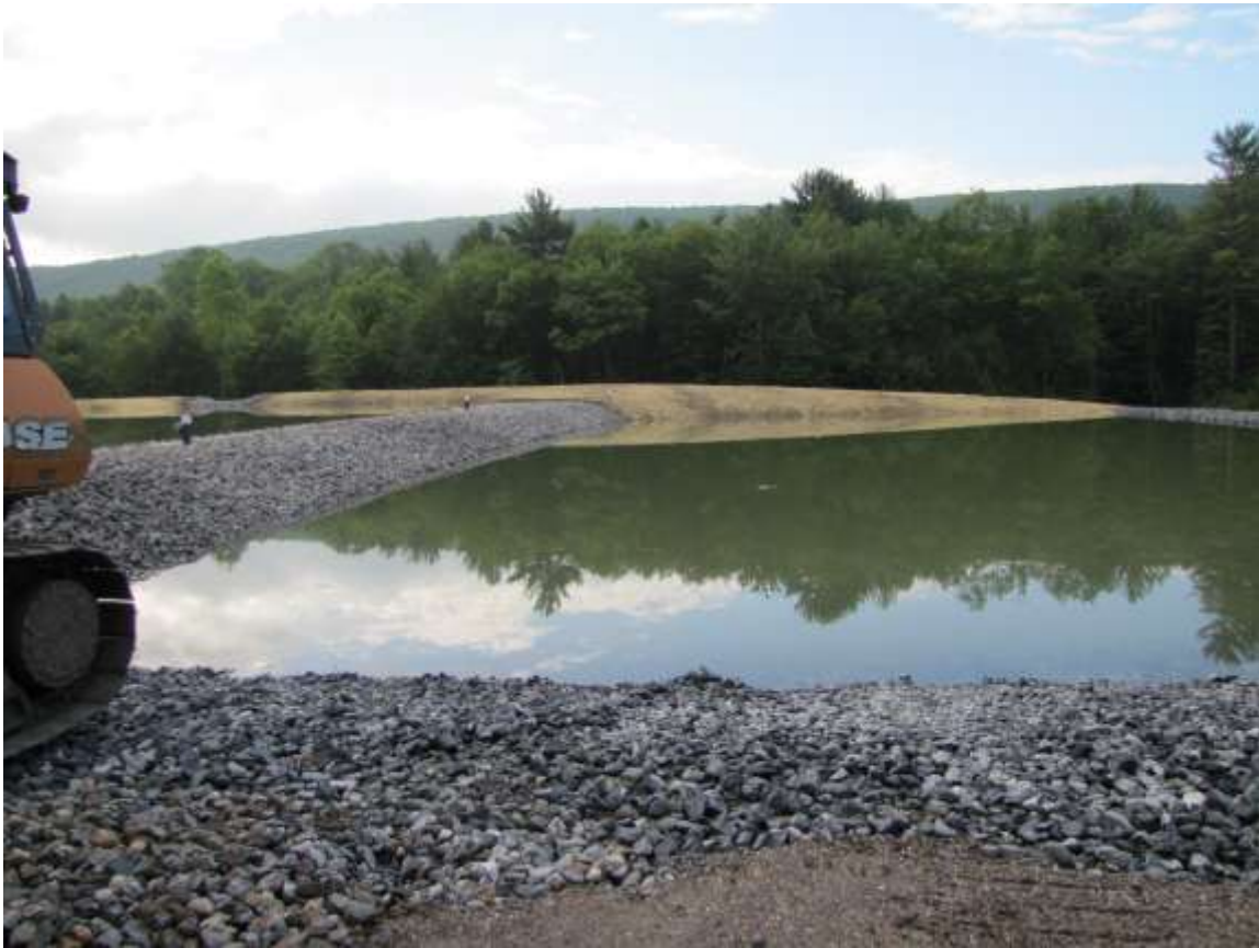
Photo 27: Treatment cell filled.
