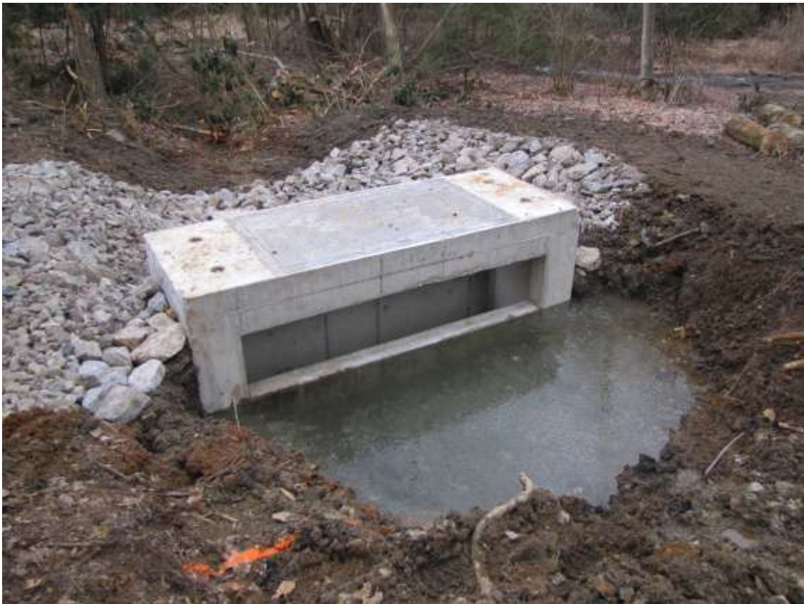
Photo 10: Intake structure installation.
