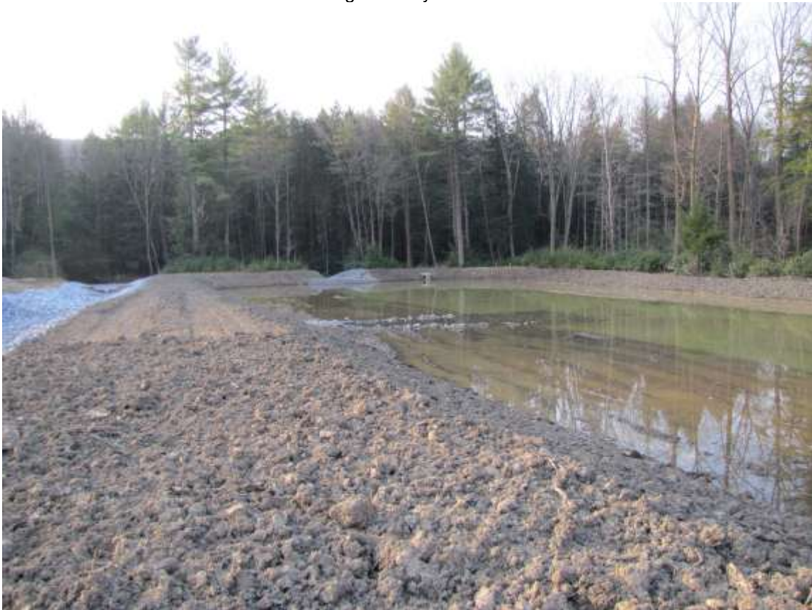
Photo 16: Completed flushing pond.
