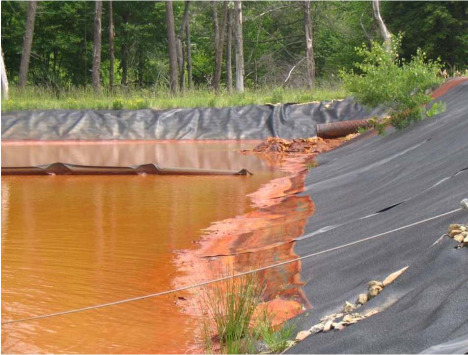
Photo C. A gap between the curtain and pond liner that allows short-circuiting. The ALD discharge pipe is in the background.
