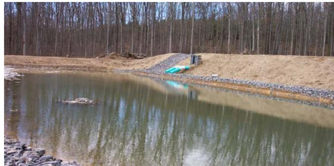
The North Branch Robbins Hollow passive treatment system has been successfully treating AMD with high acidity, high aluminum, and high iron since going online in 2004. Maintenance in the form of replenishing the organic compost (with limestone fines) and washing the limestone in the two vertical flow ponds was conducted in 2012 as preventative maintenance to ensure the continued performance of the system.
