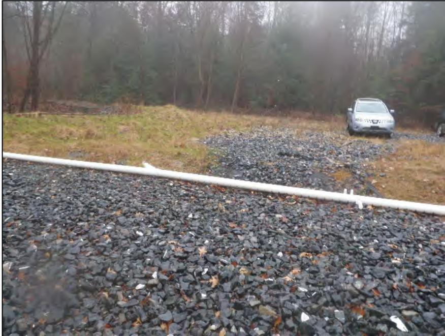
View of the inlet distribution pipe (Top) and of the entire Weaver Run D8A limestone bed (Bottom).
