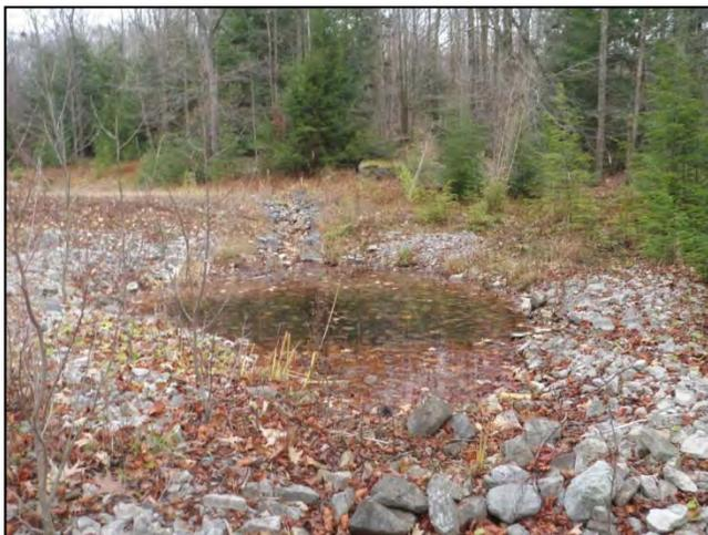
At the Bear Rock Run System 2, a limestone channel (Top Left) conveys the mine drainage to the passive treatment system. The water flows into a shallow settling pond/wetland (Top Right) and then into a limestone lined pond (Left). The water is flowing on top of the limestone-lined pond, which may indicate that the stone is plugged and needs to be cleaned.
