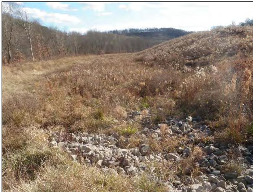
At the Reeds Run project, any remaining coal refuse that was not marketable was covered and revegetated (Top). In addition, a wetland was constructed including vegetated areas (Top) and open water habitat (Bottom). The wetland was to provide water treatment of seeps located within the project area before discharging to Reeds Run.
