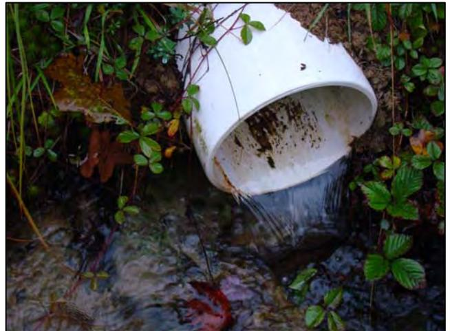
A concrete inlet box with a mesh screen is used to capture a portion of the water flowing in Shingle Run (Top Left) and then is conveyed to a buried limestone drain (Bottom Left). The effluent then discharges back to Shingle Run further downstream (Bottom Right). The mesh screen is designed to prevent rock and debris from entering the system, but at times becomes clogged (Top Right). Regular inspections and cleaning are necessary to ensure sufficient water is entering the system.
