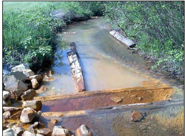
At the Neal Run site, three OPCs (Top Left) were installed as part of a coal refuse removal project to treat an extremely polluted mine discharge. While the OPCs have been very successful at removing a lot of iron in a short period of time (Top Right and Bottom Left) the water is still extremely polluted and significantly impacts Neal Run (Bottom Right). Additional treatment is needed. SRI and AWARE are currently seeking funds to expand the treatment system.
