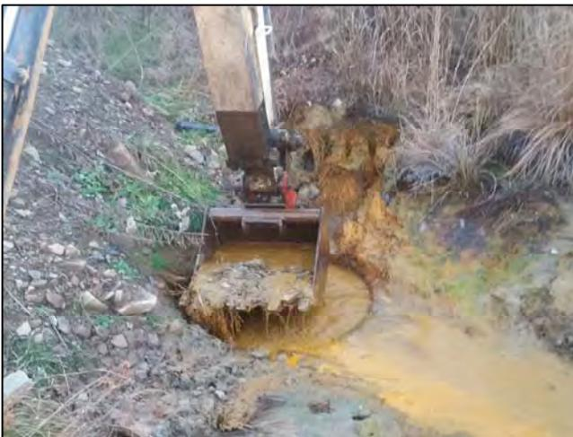
Water within the drop inlet box had to be pumped in order to access and clean the box (Top Left). The conveyance pipe to the treatment system was plugged (Top Right) as well as the piping from the flow splitter box to two of the VFRs. These were cleaned out using a power snake (Center Left). Debris that had accumulated with the mine discharge pipe was also removed (Center Right). Seeps from the leaking Settling Pond and potential other sources flow into South Branch Two Lick Creek (Bottom Left).
