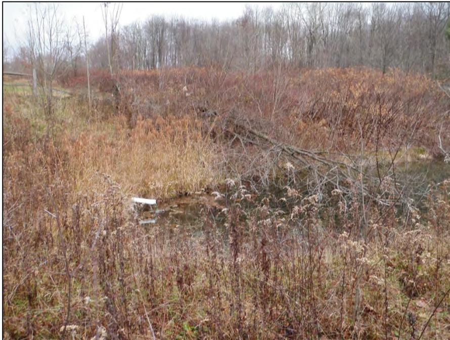
At the Gray Run passive system, fencing, downed trees, thick thorny vegetation, etc., made traveling around and seeing the system difficult. The system which is nearly 20 years old consists of a SAP or VFP (Top) and a settling pond (Bottom) which are not fully treating the water.
