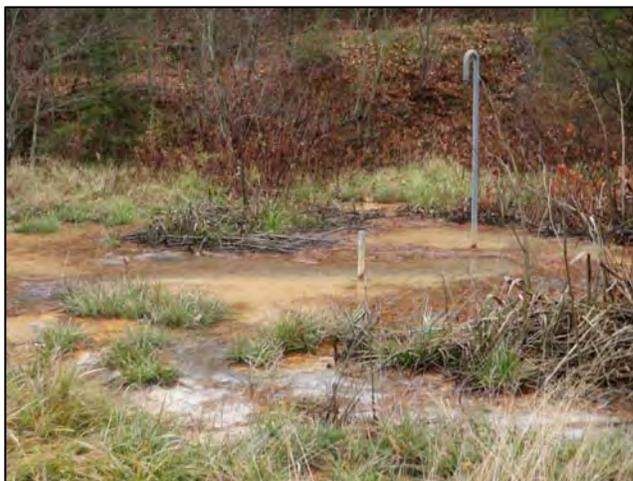
The Jamison Borehole discharge (Top Left) on this day was being controlled and the flow rate significantly reduced, which caused most of the flow to emanate at an old airshaft (Bottom Right). Under normal flow conditions, the AMD enters three settling ponds (Top Right and Bottom Left) which are undersized and do not have an alkalinity-generating component, allowing for little treatment to occur.
