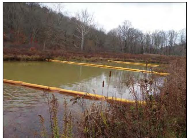
At the Kolb passive system, a large underground mine discharge has been collected and conveyed by pipe to two aerobic settling ponds in series. A large fountain (Left) was installed to provide aeration and degassing of CO<sub>2</sub> to promote oxidation of dissolved iron, while baffle curtains (Right) were installed to help settle solids. The treatment system would benefit from being expanded to include a constructed wetland and using persistent vegetation.
