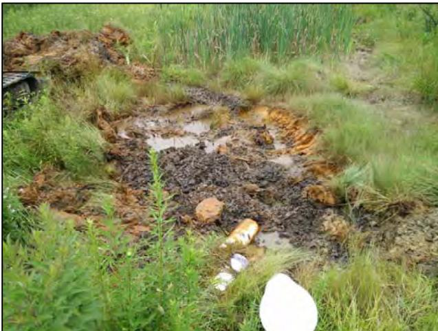
The permeability of the Coal Pit Upper Vertical Flow Pond had decreased and was flowing over the berm (Top Left). The pond was drained and stirred (Top Right). The valve for flushing the pond had broken and was replaced (Middle Left). Vegetation, sludge, and debris had accumulated around the influent pipe of the Lower system (Middle Right) which made sampling difficult. The material was removed (Bottom Left).
