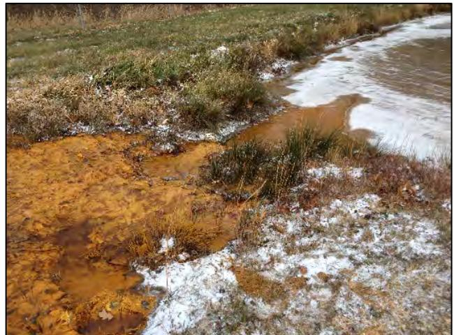
At the Jenners passive system, the AMD emanates from an old municipal water supply well (Top Left). A build up of iron sludge and failing wooden baffles may be causing short-circuiting within the first settling/aeration pond (Top Right and Bottom Left). The wooden baffles could be replaced with directional curtain baffles. Iron precipitates within the spillway between the first settling/ aeration pond and the vertical flow pond (Bottom Right) are likely increasing water levels within the ponds.
