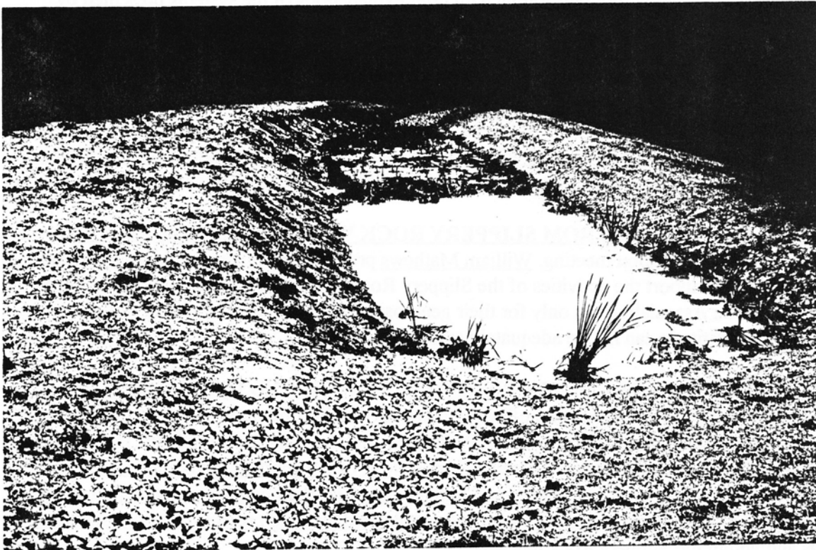
Pond/Wetland for recently completed vertical flow system at SR 109, PA Gamelands No. 95
