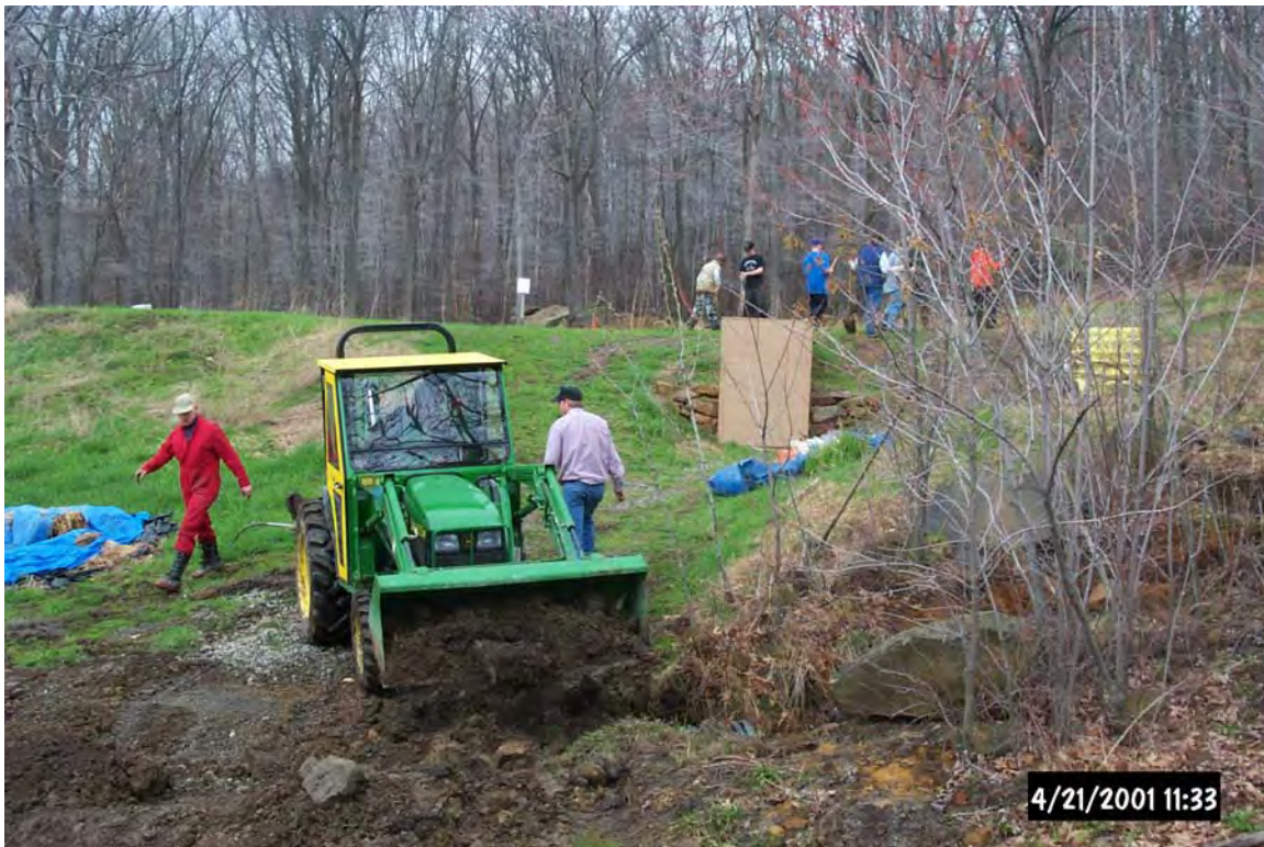
Maintenance being conducted by volunteers during Jennings's "Spring into Action Day" .
