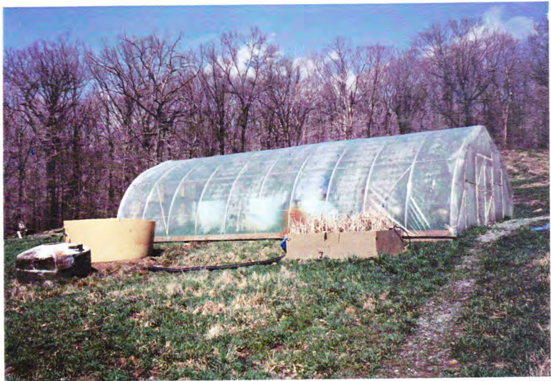
QUONSET HUT, TEST BED WETLANDS AND PILOT-SCALE TANKS are part of the on-going educational and scientific efforts at the Jennings Environmental Education Center. The quonset hut allows for demonstration systems to be evaluated year-round.
