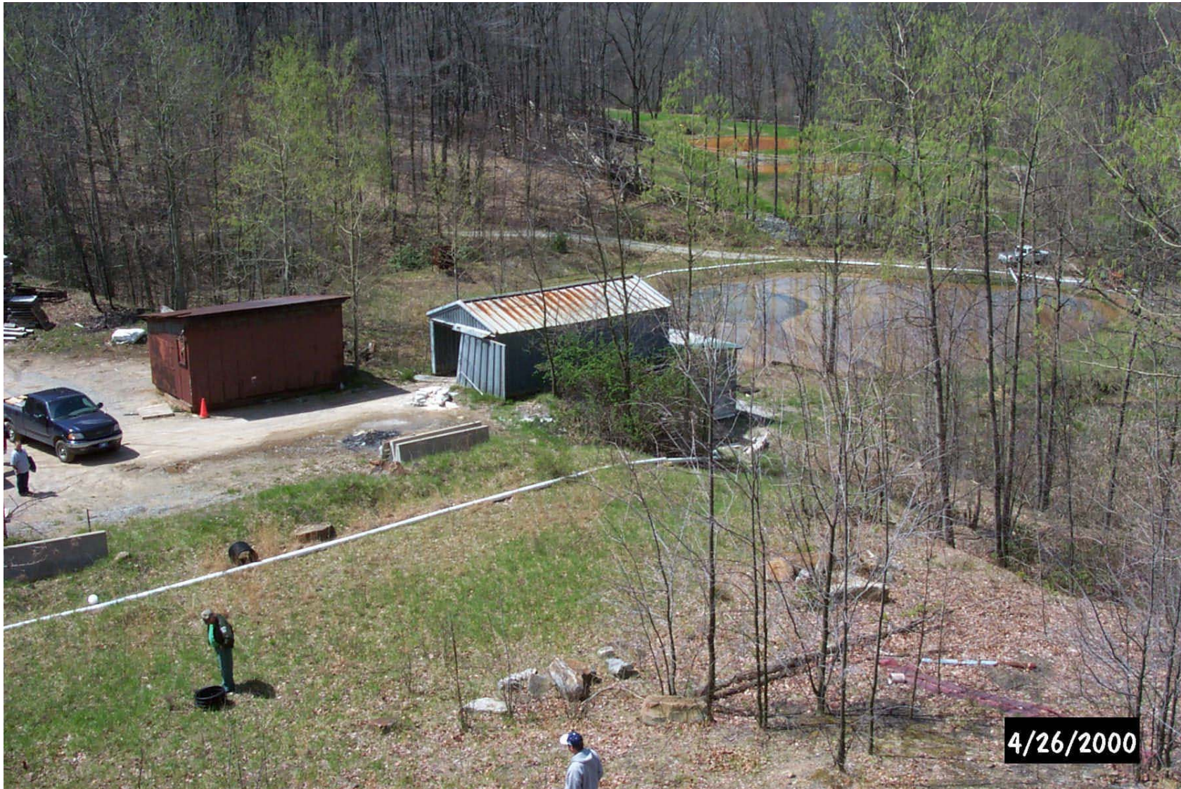
A view of the lime plant and one of the sludge ponds (Center) of the previous active system to treat the A/C discharge at Ohiopyle State Park. A portion of the Harbison Walker Restoration Area Phase I passive treatment system can be seen in the background.
