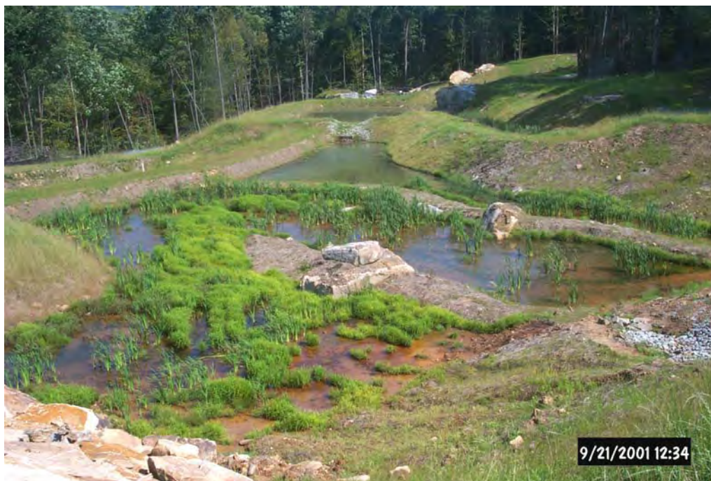
View of the Harbison Walker Phase II passive treatment system with the B1B3 Settling Pond/Wetland (foreground) and the B1B3 Vertical Flow Pond (upper center).
