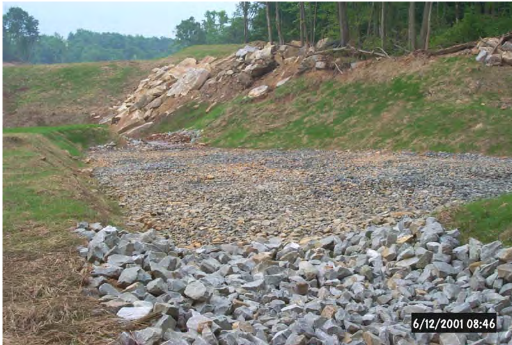
The effluent of the B1B3 Vertical Flow Pond flows through the B1B3 Settling Pond/Wetland before entering the Horizontal Flow Limestone Bed (above).
