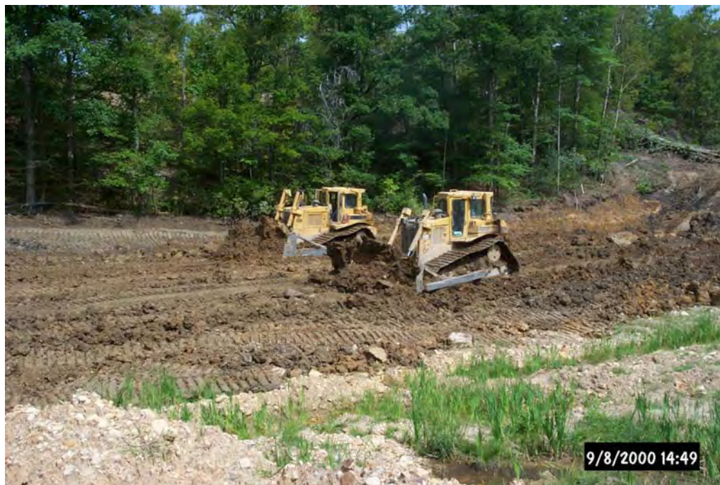
Construction of the A/C Vertical Flow Ponds by Amerikohl Mining, Inc.
