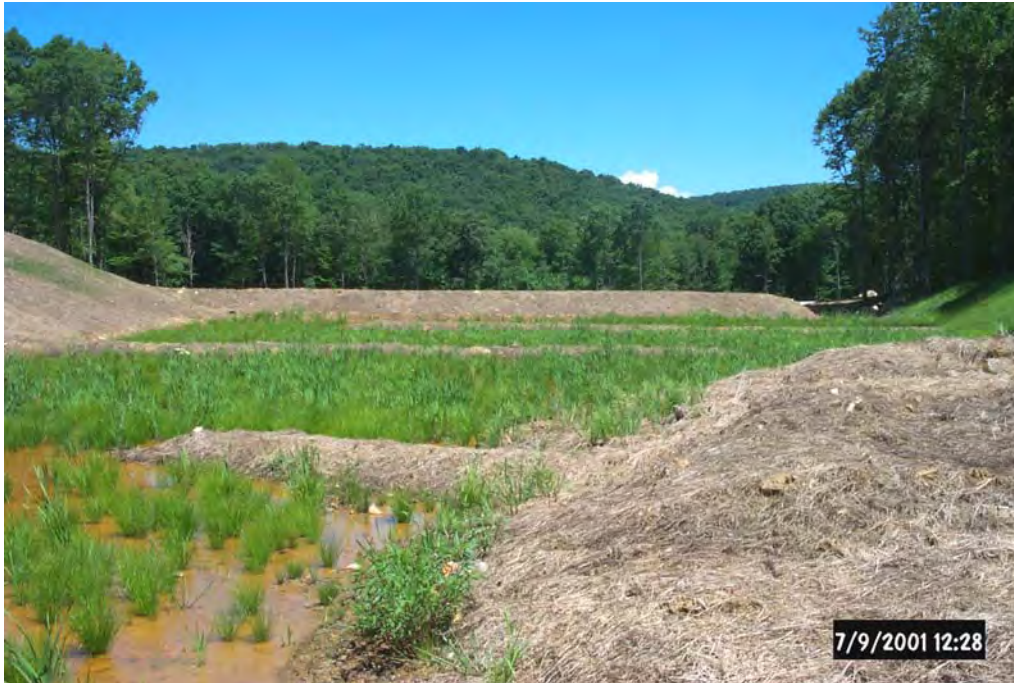
B1 Wetland #1 provides further oxidation and settling of solids following the B1 Settling Pond.
