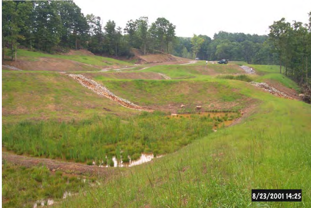
View of the Harbison Walker Phase II passive treatment system looking south towards the top of the system. B1 Wetland #1 is in the foreground. B1 Settling pond is top left.
