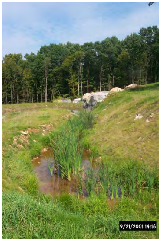
The B1 Wetland 2 and 3 are channel wetlands (bioswales) that convey the flow of the B1 discharge into the B1B3 Vertical Flow Pond that provides treatment of the B1 discharge as well as the B3 discharge.
