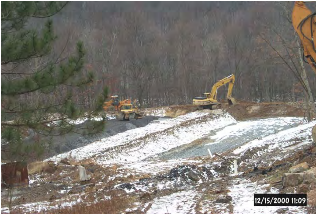
View of the construction of the A/C Vertical Flow Ponds.
