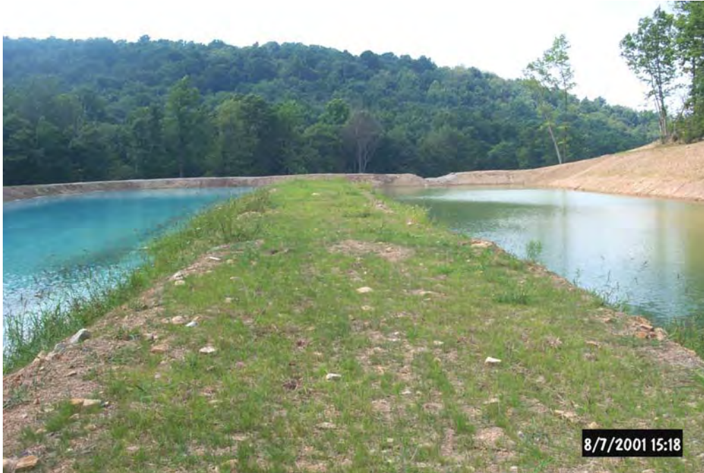
Completed A/C Vertical Flow Ponds North (right) and South (left)
