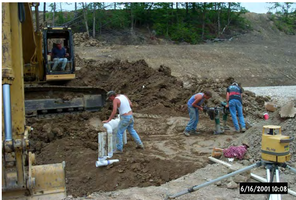
Replacement of a portion of the piping system of the A/C Vertical Flow Pond by Amerikohl Mining, Inc. as part of the maintenance agreement.
