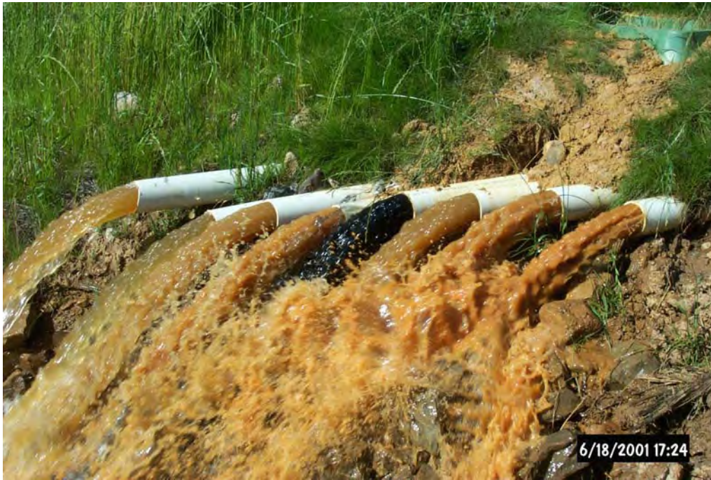
Flushing of the B1B3 Vertical Flow Pond. Note the thick, dark orange-colored, iron-bearing, water.
