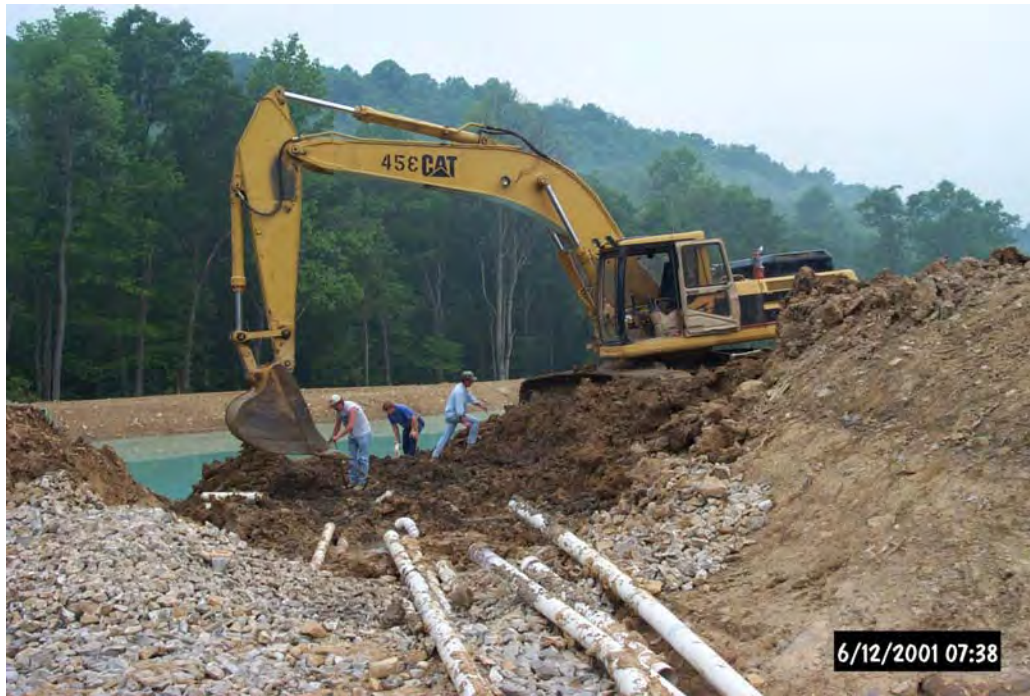
Replacement of a portion of the piping system of the A/C Vertical Flow Pond by Amerikohl Mining, Inc. as part of the maintenance agreement.
