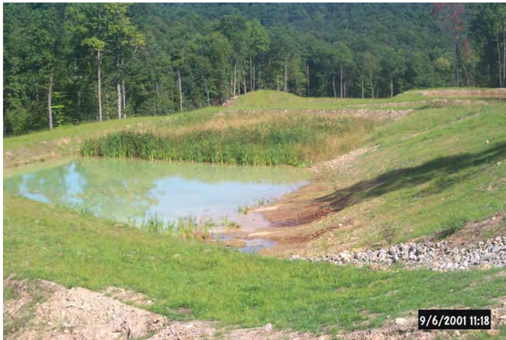
After discharging from the A/C Vertical Flow Ponds, the water flows through a riprap channel into the A/C Settling Pond/Wetland.
