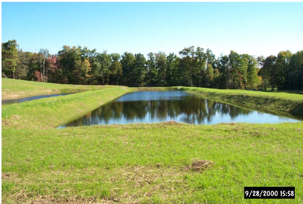
View of De Sale Phase II Vertical Flow Pond West (Center) and Vertical Flow Pond East (Far Left).
