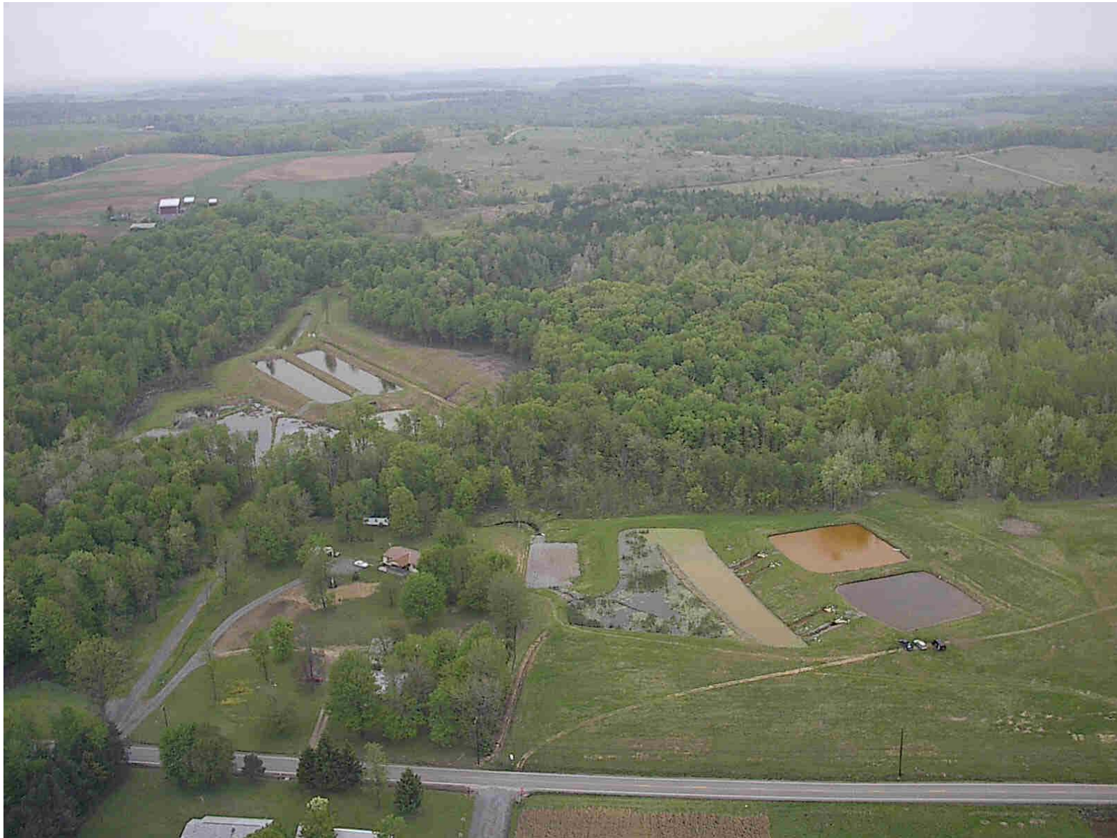
Ariel view of the De Sale Restoration Area. The Phase I passive treatment system is on the right while the Phase II passive treatment system is on the left.
