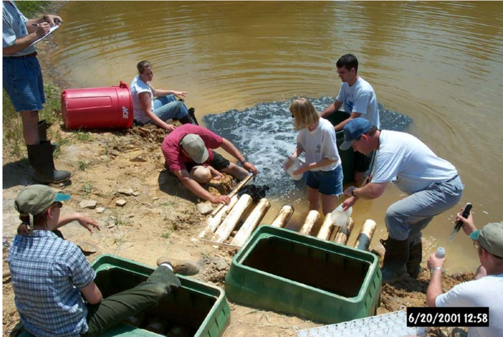
Each pipe discharges from one of eight quadrants within the Vertical Flow Pond. Note the black coloring of the flush water.
