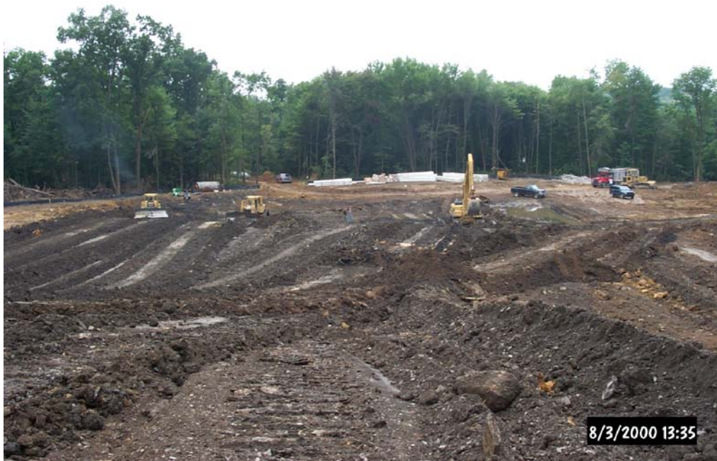
Construction of the De Sale Phase II Passive Treatment System.
