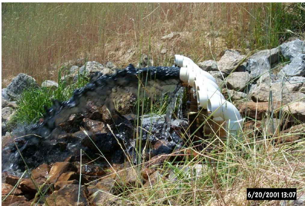
Each pipe discharges from one of eight quadrants within the Vertical Flow Pond. Note the black coloring of the flush water.
