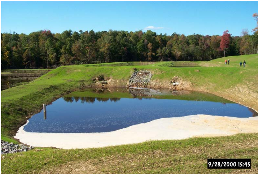
The Settling Pond receives the effluent from the Vertical Flow Ponds and is also used as a flush pond.
