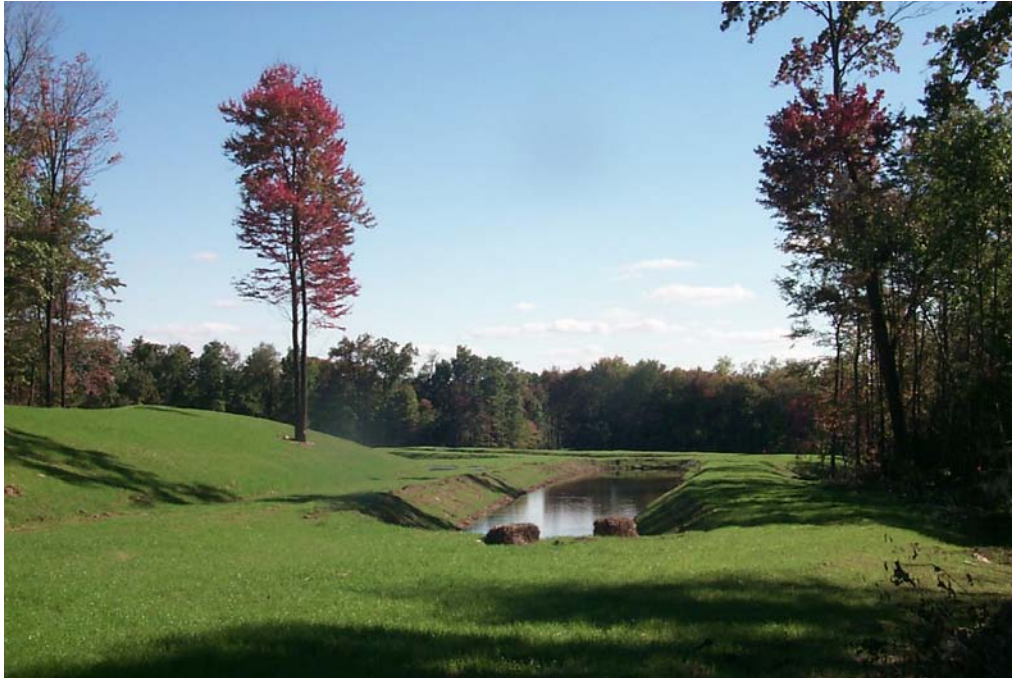
View of the De Sale Phase II Forebay looking towards the passive system.
