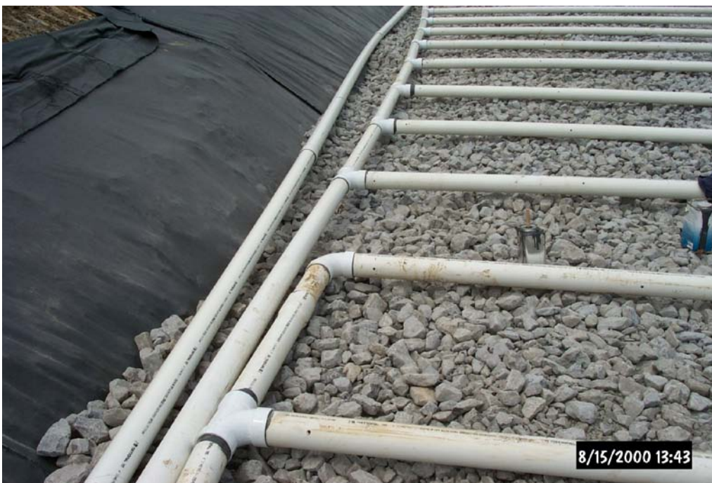
Construction of the underdrain piping system for Vertical Flow Pond East by Amerikohl Mining Inc., employees.
