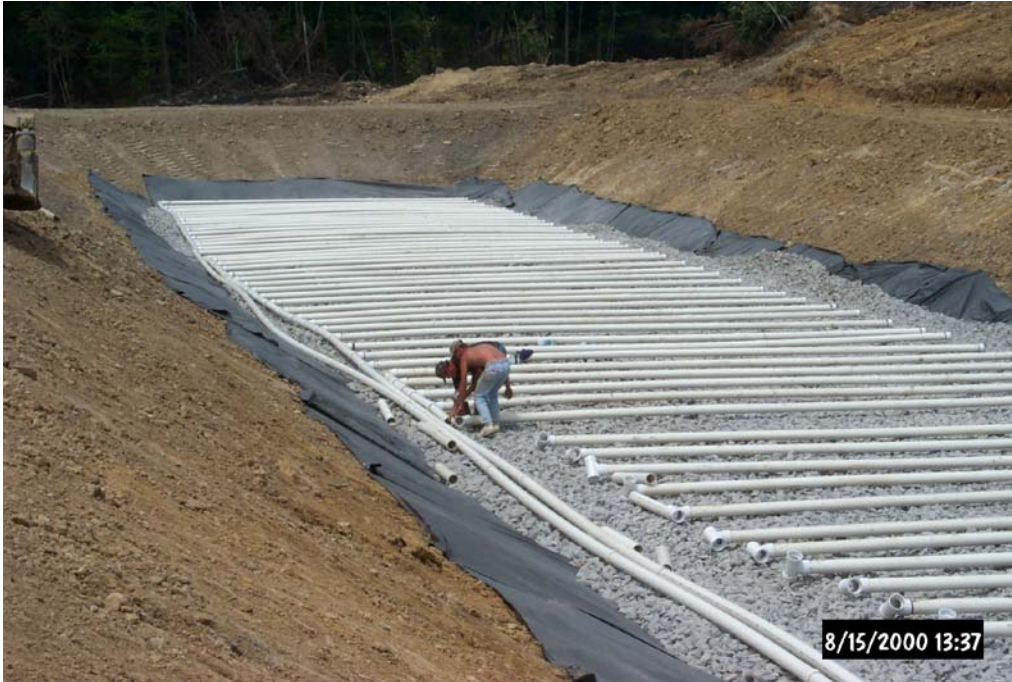
Construction of the underdrain piping system for Vertical Flow Pond East by Amerikohl Mining Inc., employees.
