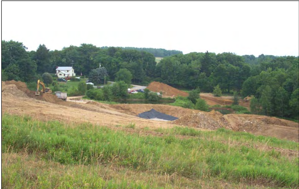
View of the De Sale Phase III passive system under construction ( Above ). To the left, an excavator is digging the collection ditch. In the center is Vertical Flow Pond 1. To the right is a dozer constructing the basin for the Horizontal Flow Limestone Bed. During construction several unknown buried pipes were discovered ( Below ).
