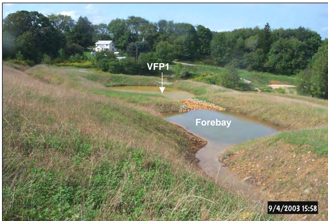
View of the completed De Sale Phase III passive treatment system, which incorporated three previously existing ponds in the design.
