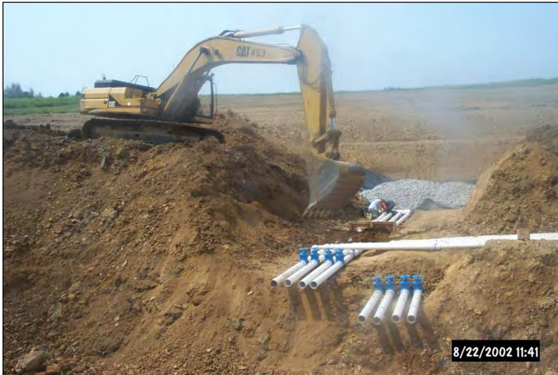
Installation of the Vertical Flow Pond 1 flush pipes.
