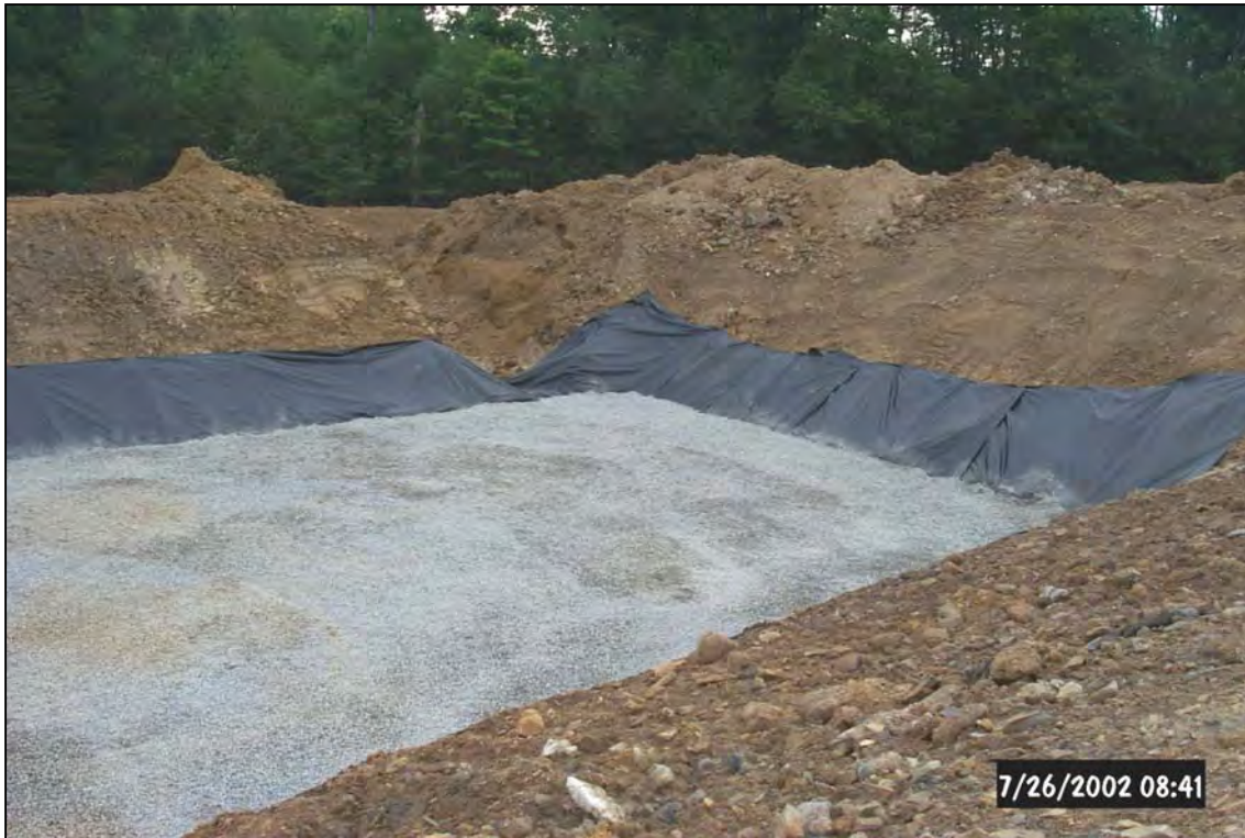
The lower tier of pipes were bedded in stone in Vertical Flow Pond 1 (Above) . Construction of the basin for the Horizontal Flow Limestone Bed (Below) .
