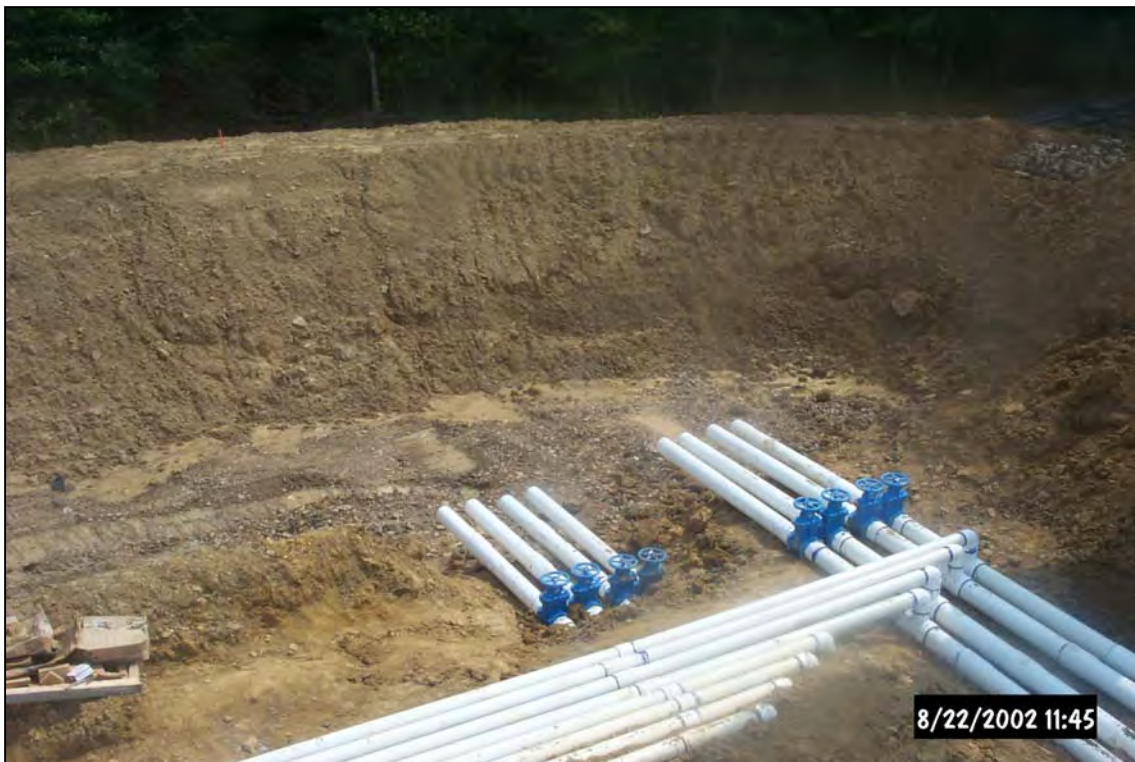
Installation of the Vertical Flow Pond 1 flush pipes.
