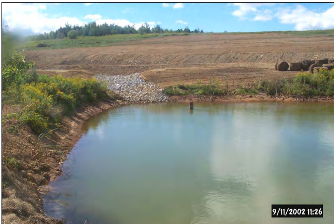
View of the forebay and a portion of the collection ditch during installation of the flushing pipes of Vertical Flow Pond 1 (Above) . The sludge drying beds on top of the hill were reclaimed and the land returned to approximate original contours (Below) .
