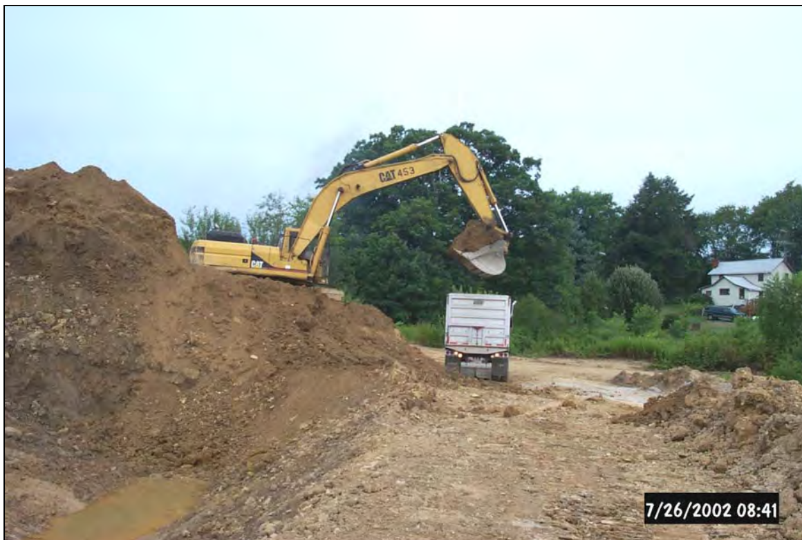
The passive treatment system was designed by BioMost, Inc., and constructed by Amerikohl Mining, Inc. The installation of the collection ditch can be seen in both the top and bottom photos.
