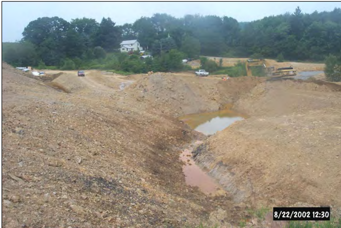
View of the forebay and a portion of the collection ditch during installation of the flushing pipes of Vertical Flow Pond 1 (Above) . The sludge drying beds on top of the hill were reclaimed and the land returned to approximate original contours (Below) .
