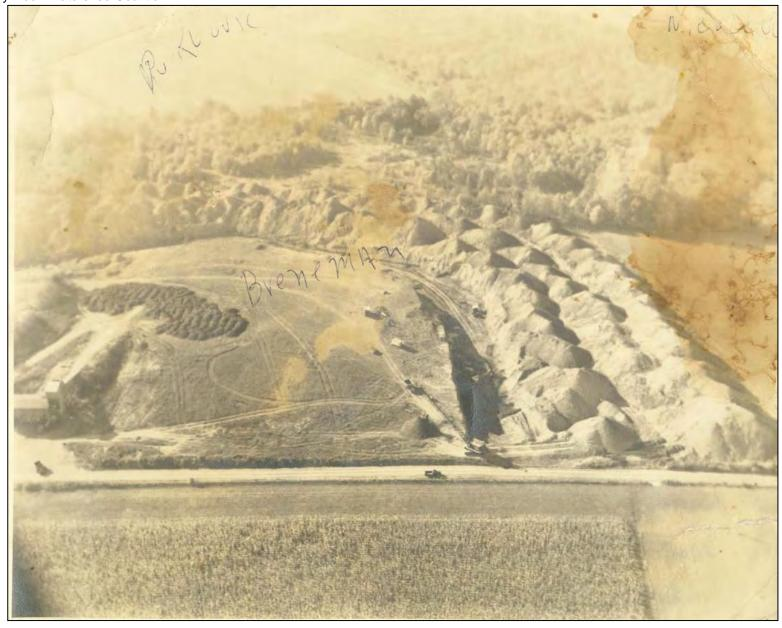
"Aerial" photograph of the original mining (Circa 1940's). The dragline (near the center), working pit and surrounding spoil piles can be seen. The site was left unreclaimed except for planting trees on the spoil.
