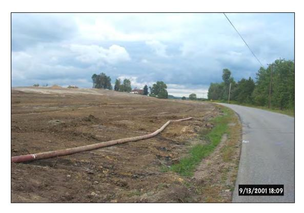
As part of the reclamation process, the acidic, abandoned mine drainage in the open pits was pumped to treatment ponds and chemically treated before discharging to an unnamed tributary to Wolf Creek.
