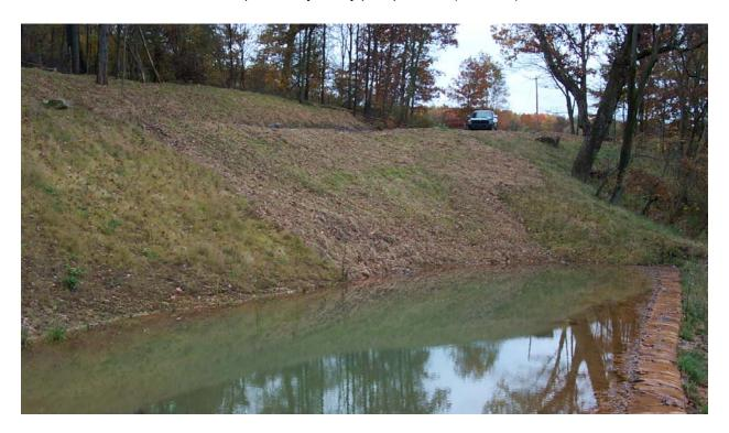
OSM Funding was used to install a French drain upgradient of the cut slope to intercept the subsurface flow, install buried limestone riprap reinforcement and successfully stabilize the slope. (10/20/04)
