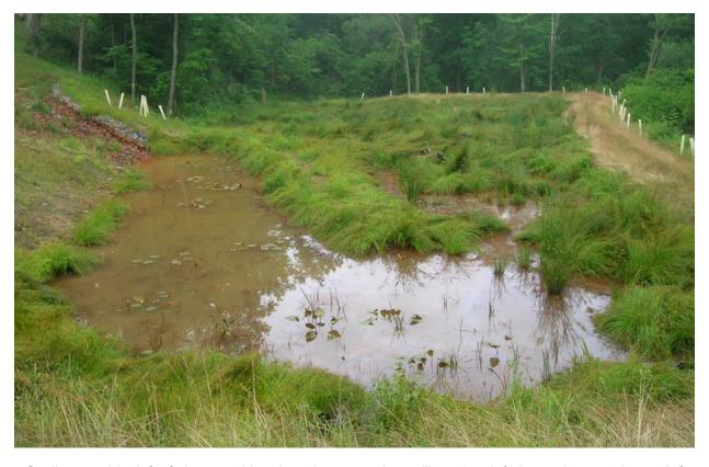
Settling pond (to left of photograph) outlets via an aeration spillway (top left) into a drop pond area (left and foreground), flows into the aerobic wetland and outlets to Semiconon Run near the top center of the photograph. System currently reduces iron concentrations from 22 mg/l to less than 3 mg/l.
