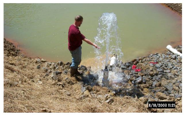
After the initial buried collection systems were installed, the discharge was successfully collected and directed into the passive system. Vigorous agitation and aeration was achieved using the available hydraulic gradient. The system functioned very well through the fall of 2003.
