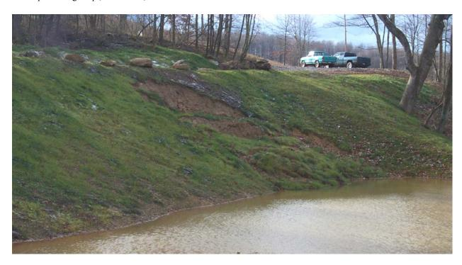
Slumping occurred above the settling pond due to significant shallow subsurface flows that were likely exasperated by heavy precipitation. (11/13/03)
