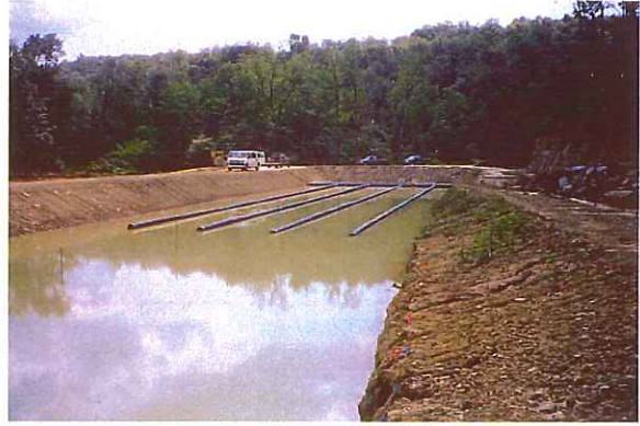
Limestone Pond prior to limestone placement. Flushing network is visible.
