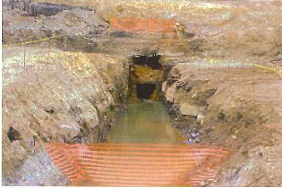
Excavated drainage heading.
