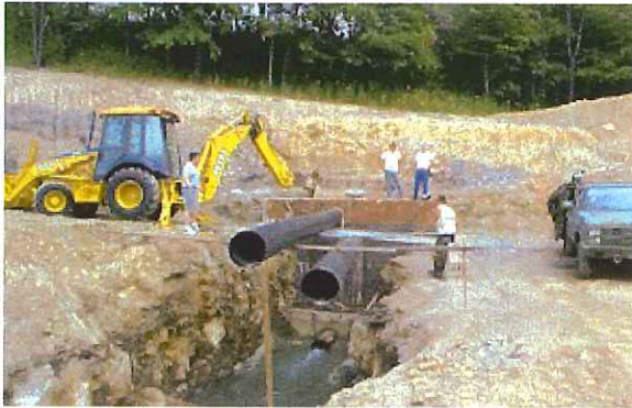
Pipe being fitted to storm water control structure.
