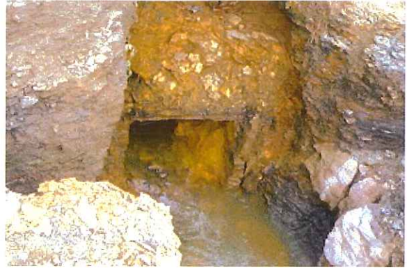
Closeup view of exposed drainage heading.
