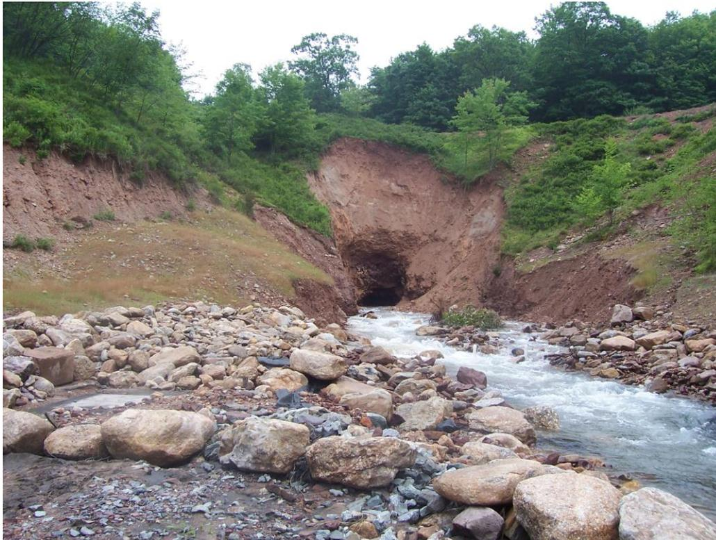
Picture 13. Damage to intake system and mine opening during the June 2006 flooding.
