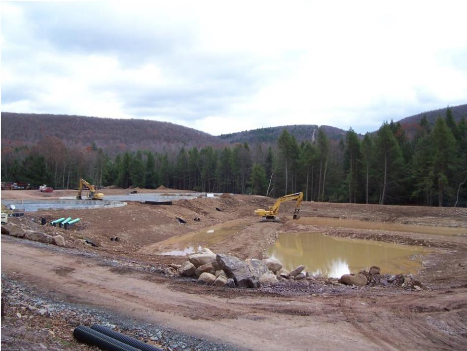
Picture 9. View of first settling pond before stabilization and berm construction was completed.
