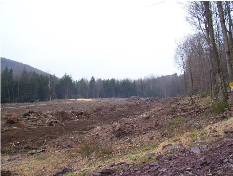
Picture 5. Limestone tank and settling pond site preparation through clearing and grubbing .
