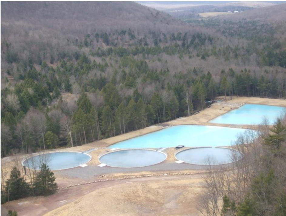
Picture 11. Aerial view of limestone tanks, and two settling ponds while system was in operation.
