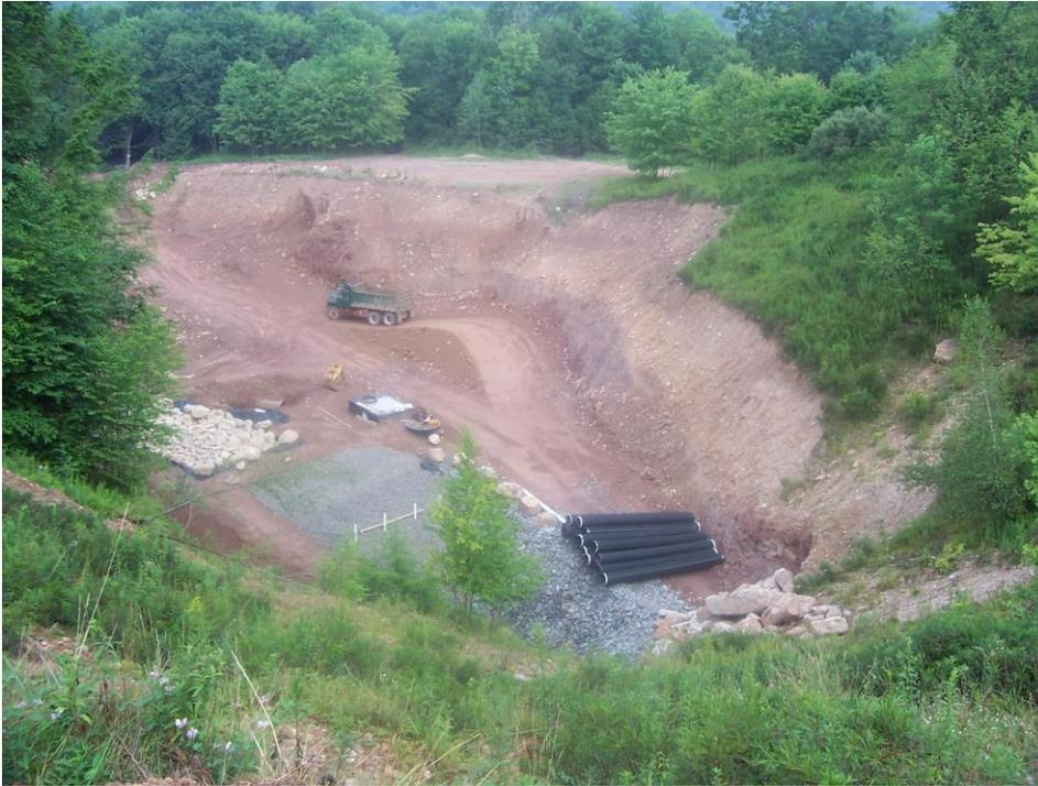
Picture 4. View from above the Audenreid mine tunnel opening showing the completed rock filter, rip-rap lined overflow channel and cleared mine opening with water being diverted around the intake system.
