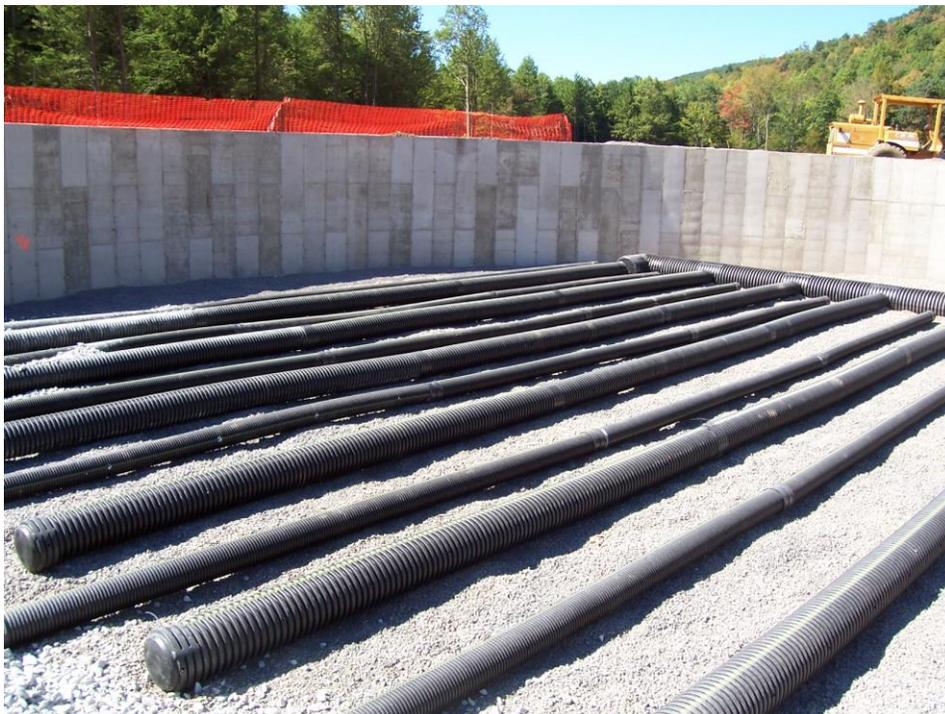
Picture 7. View perforated pipes on top of non calcareous rock bed for the flushing system piping (large diameter pipes) and water intake piping (small diameter pipe) in the limestone tanks.
