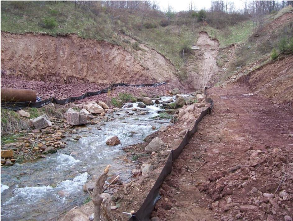
Picture 2. Preparing the mine opening and surrounding area for intake system with proper E&S controls being utilized.
