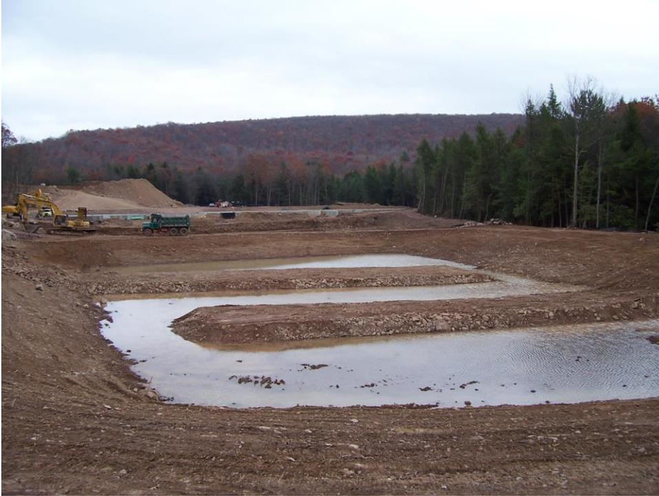
Picture 10. View of second settling pond before bank stabilization.
