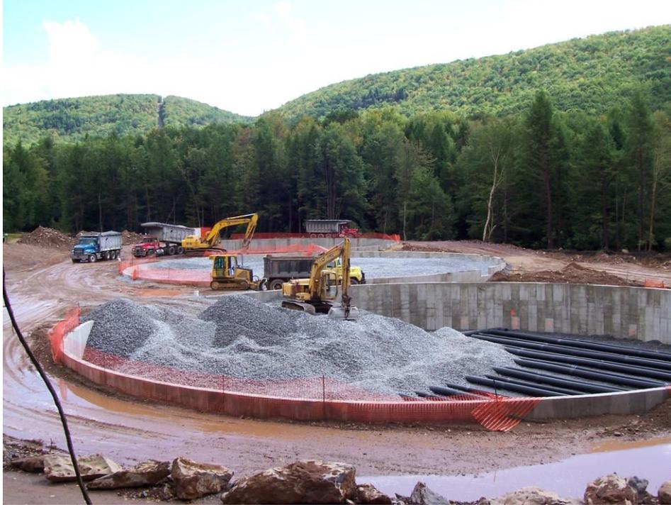
Picture 8. Limestone additions to tanks.
