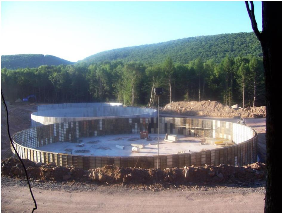
Picture 6. View of two completed concrete limestone tanks in background while recently poured concrete is “setting up” in tank mould in the foreground.
