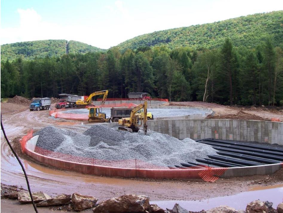
Picture 8. Limestone additions to tanks.
