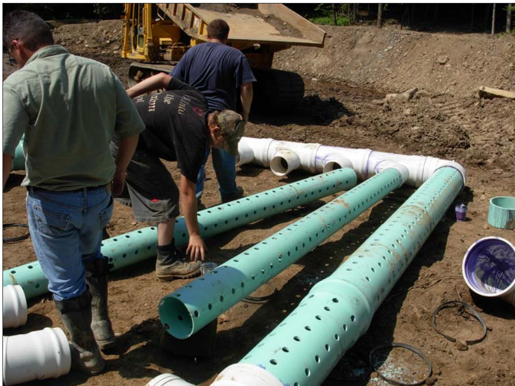
Assembling the Intake Manifold to capture and convey the 87-2 discharge under Fox Run to the passive system (Summer 2008).
