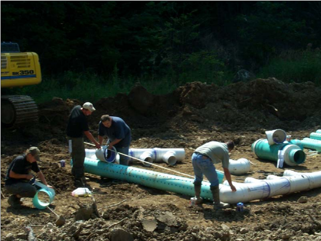
Assembling the Intake Manifold to capture and convey the 87-2 discharge under Fox Run to the passive system (Summer 2008).
