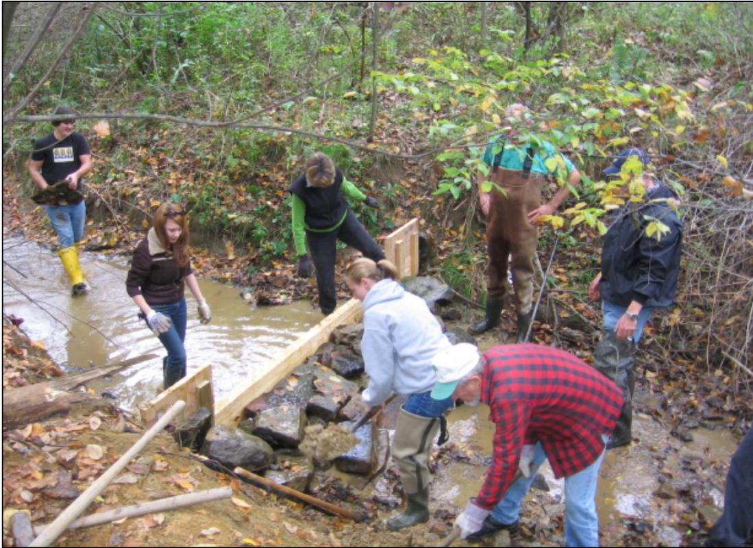
Students from the Indiana University of PA and volunteers from AWARE help to construct a weir on Reeds Run at sample point 851-2. Only three of the four weirs could be constructed due to the damming of the water.
