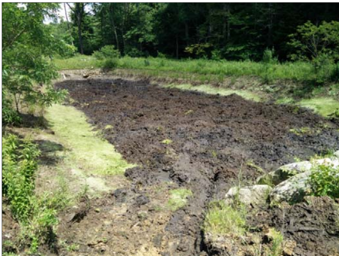
Top Left: The Vertical Flow Pond of the Upper System had become plugged and at times a large portion of the water was flowing through the emergency spillway. Right: During the site visit, the flush valve was opened with difficulty, but the VFP drained very slowly indicating that permeability of the treatment media had significantly decreased and likely the cause of the problem. Bottom Left: Once drained, the vertical flow pond was stirred to restore full flow through the system components.
