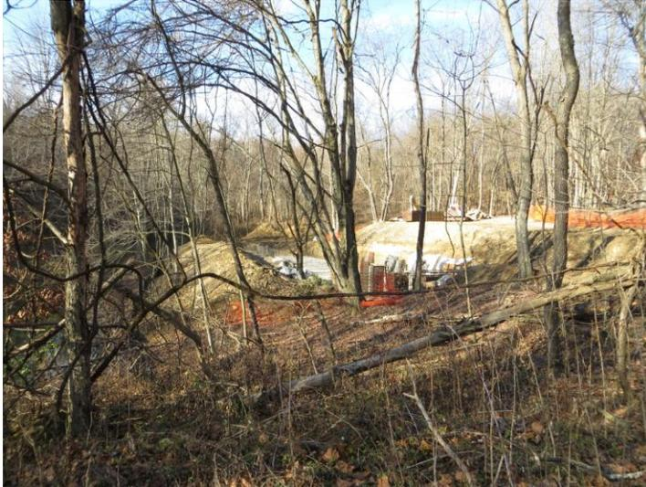
The DLB system is not quite complete. The concrete work is done but the 450 tons of limestone aggregate has not been delivered due to the weather. The bed is 4.5 ft deep and approximately 20 ft. by 100 ft. The sizing is based on the highly conservative assumption of 15 gpm flow and acidity removal. This conservative design was utilized so that its effectiveness will be assured and so that cleaning of the limestone should only be necessary every 10 years.
