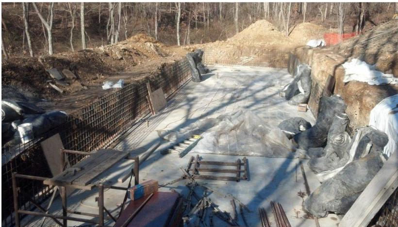
The DLB is a 4.5 ft thick bed of limestone aggregate and does not contain any organic matter. The bed is completely flooded during routine operation, but there is no need for standing water on top of the stone. Aluminum solids accumulate in the limestone aggregate. The deleterious effect of the solids is mitigated by rapidly draining the bed empty every week. The
