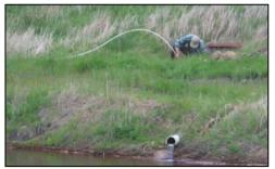
need to be cleaned out when the capacity is reduced by 25 percent. Cleanouts for the anoxic collection systems may need to be periodically used to keep the pipes clear. Cleaning pipes can be carried out by using pipe clean-out rods, industrial snake clean-out tools, backflushing, or other reasonable methods.
