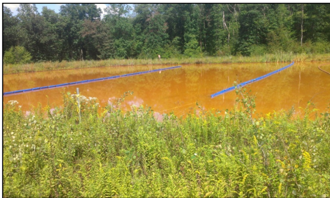
At the Erico Bridge PTS, water was discharging over the HFLB emergency spillway ( top left ) indicating either the piping or limestone aggregate was plugged. In addition, beaver had built a dam across the spillway ( top left ) causing the water level within the treatment wetland to rise and, in places, flow over the berm, flooding the access road ( top right ). The HFLB pipe was back-flushed ( center ) using an air compressor ( middle left ). New baffle curtains were also installed ( middle right ) in Settling Pond 1 ( bottom left ) and Settling Pond 3 ( bottom right ).
