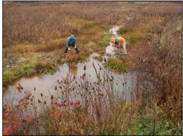
Channelization within the treatment wetland (*top left*) of the SR-286 PTS is apparently in response to the uneven build-up of vegetation within the forebay level spreader. Volunteers helped to replace rocks and to remove vegetation in order to re-establish the level spreader (*top right*). Compost filter socks were installed to replace the hay bales that had been previously installed in 2004 to increase storage capacity of the wetland and to reduce short-circuiting (*bottom left & right*).
