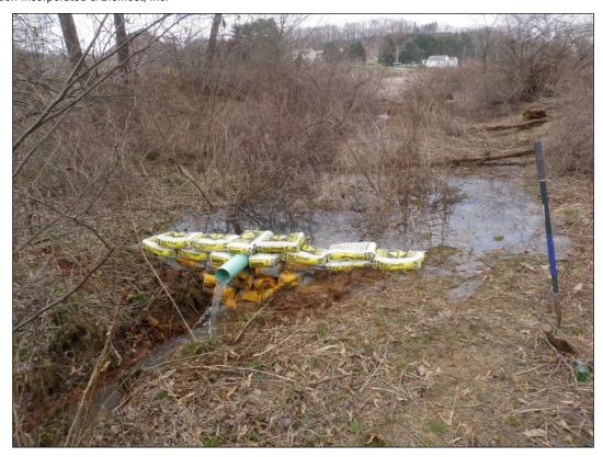
Concrete bags, with bentonite used to seal void spaces between bags, were used on 4/9/13 to protect the existing wetland channel outlet replacement pipe (above). On 6/17/13, outlet pipe remained in place and water level had risen (below).
