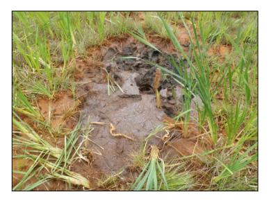
The bacteria *Gallionella* is growing and clogging the limestone aggregate within the Oxic Limestone Drain causing the water to rise to the surface and flow over top of the system *(top left & right)* and then flow over the spillway *(bottom left)* into the next pond instead of through the OLD. This problem requires flushing of the bed *(bottom right)* on an essentially weekly basis which is quite time consuming.
