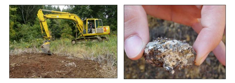
The Pittsburgh Airport Authority provided an excavator and operator to stir the treatment media within the VFPs (Left). Unfortunately because of the piping system, only the top foot of material could be stirred. Aluminum solids coated the limestone of the Upper VFP (Right). There will likely be a need to reevaluate this system in the near future and potentially rehabilitate the VFPS.
