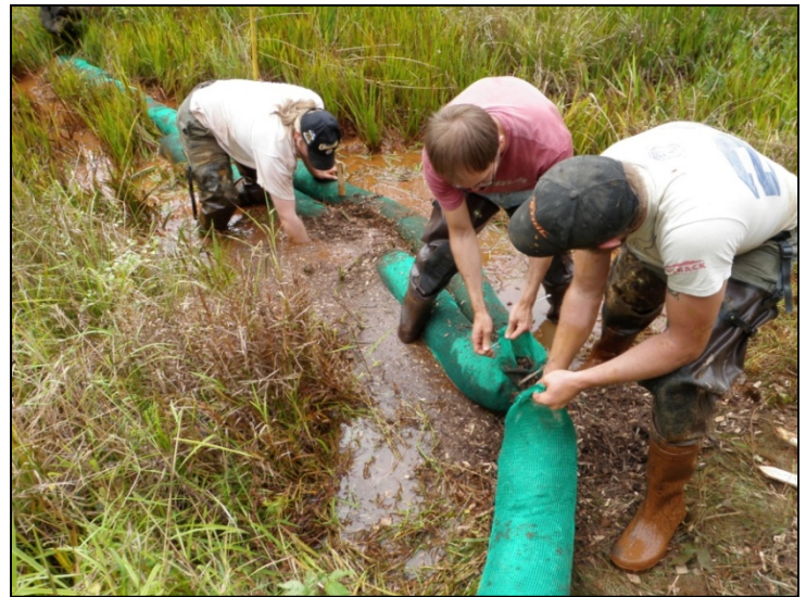
Channelization in the treatment wetland ( top left ) was causing short-circuiting to occur resulting in decreased treatment efficiency. The channelization was disrupted by installing compost filter sox ( top right and bottom right ) to block flow paths and deflect water into other underutilized areas of the treatment wetland. Iron sludge, organic debris, plants, etc., had accumulated behind the level spreaders preventing the water from being evenly distributed ( bottom left ). This area was cleaned out with much assistance provided by Camp Lutherlyn volunteers ( bottom left ).
