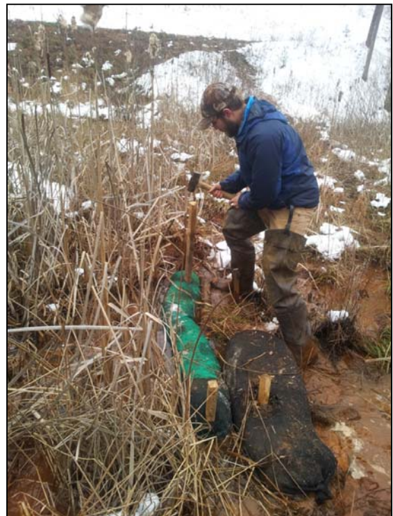
Channelization in the treatment wetland ( top left ) was causing short-circuiting to occur resulting in decreased treatment efficiency. The channelization was disrupted by installing compost filter sox ( top right and bottom right ) to block flow paths and deflect water into other underutilized areas of the treatment wetland. Iron sludge, organic debris, plants, etc., had accumulated behind the level spreaders preventing the water from being evenly distributed ( bottom left ). This area was cleaned out with much assistance provided by Camp Lutherlyn volunteers ( bottom left ).
