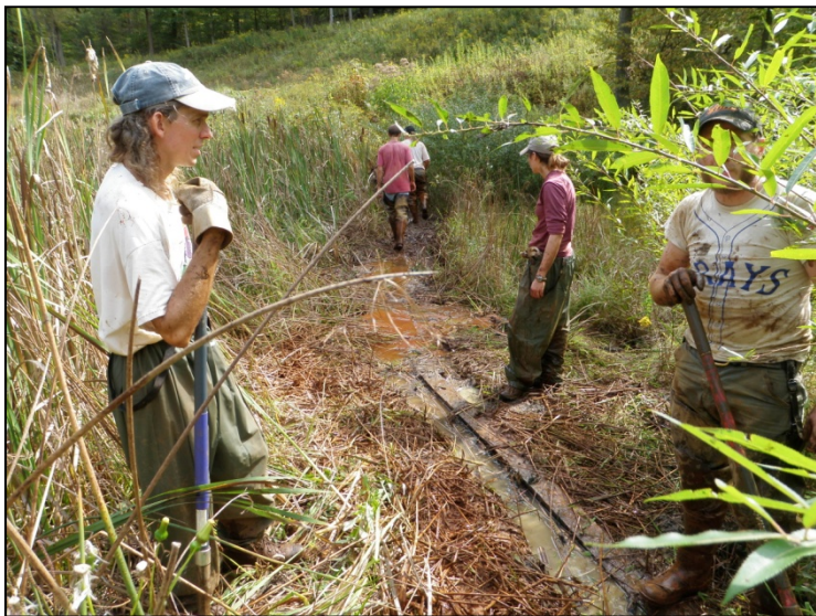
Channelization in the treatment wetland ( top left ) was causing short-circuiting to occur resulting in decreased treatment efficiency. The channelization was disrupted by installing compost filter sox ( top right and bottom right ) to block flow paths and deflect water into other underutilized areas of the treatment wetland. Iron sludge, organic debris, plants, etc., had accumulated behind the level spreaders preventing the water from being evenly distributed ( bottom left ). This area was cleaned out with much assistance provided by Camp Lutherlyn volunteers ( bottom left ).
