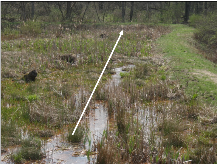
Channelization in the treatment wetland ( top left ) was causing short-circuiting to occur resulting in decreased treatment efficiency. The channelization was disrupted by installing compost filter sox ( top right and bottom right ) to block flow paths and deflect water into other underutilized areas of the treatment wetland. Iron sludge, organic debris, plants, etc., had accumulated behind the level spreaders preventing the water from being evenly distributed ( bottom left ). This area was cleaned out with much assistance provided by Camp Lutherlyn volunteers ( bottom left ).
