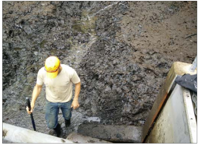
Top Left: Flushing the forebay using a pump to direct organic matter to the flush pipe. Top Right: Removing organic matter by hand. Bottom Left: The siphon vault was washed. Bottom Right: The siphons were disabled by removing a plug to allow the cyclone to function properly.
