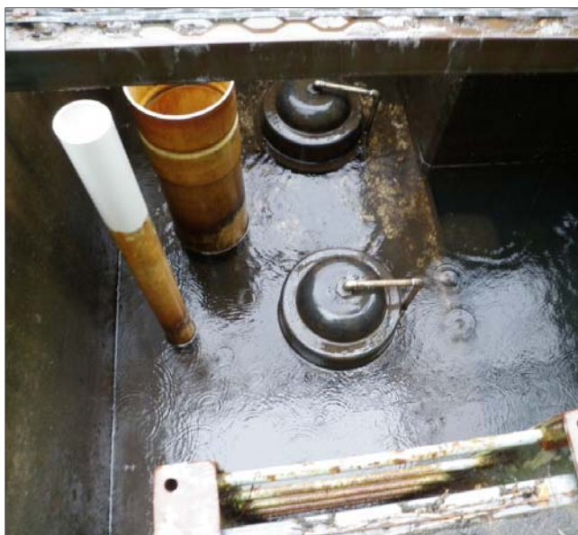
Top Left & Right: The cyclone screen being cleaned to allow flow to the Oxid Limestone Drain. Bottom Left: The siphons which may be disabled as needed to allow the cyclone to function properly. Bottom Right: The bearings for the cyclone screen were replaced.
