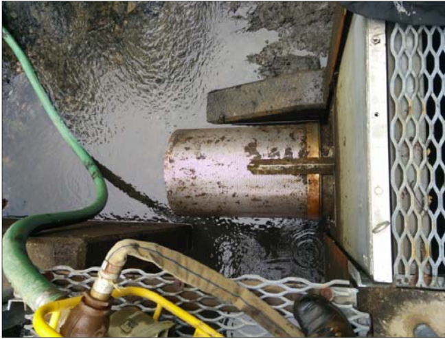
Top Left: Flushing the forebay using a pump to direct organic matter to the flush pipe. Top Right: Removing organic matter by hand. Bottom Left: The siphon vault was washed. Bottom Right: The siphons were disabled by removing a plug to allow the cyclone to function properly.
