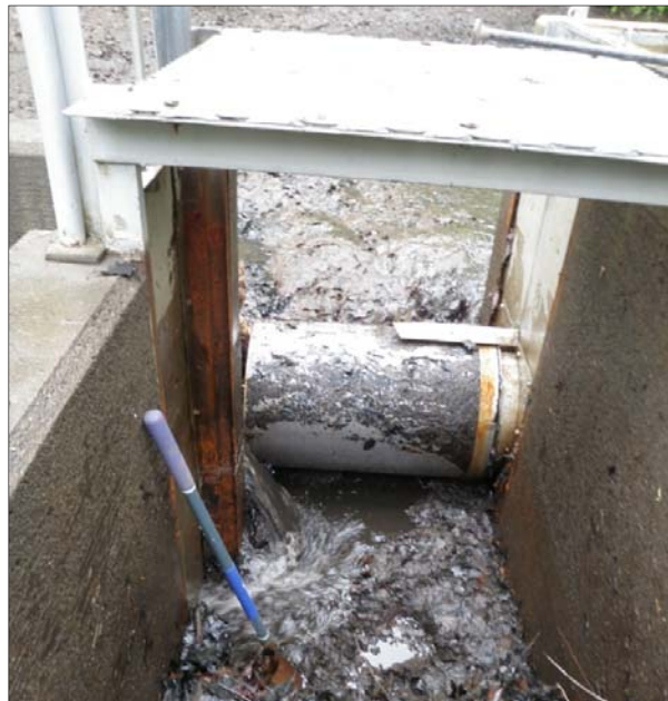
Top Left & Right: The cyclone screen being cleaned to allow flow to the Oxid Limestone Drain. Bottom Left: The siphons which may be disabled as needed to allow the cyclone to function properly. Bottom Right: The bearings for the cyclone screen were replaced.
