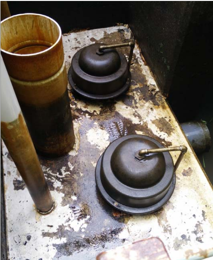
Top Left: Flushing the forebay using a pump to direct organic matter to the flush pipe. Top Right: Removing organic matter by hand. Bottom Left: The siphon vault was washed. Bottom Right: The siphons were disabled by removing a plug to allow the cyclone to function properly.
